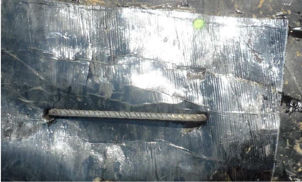
Figura4: Mechanical fixation of the geosynthetic colth
