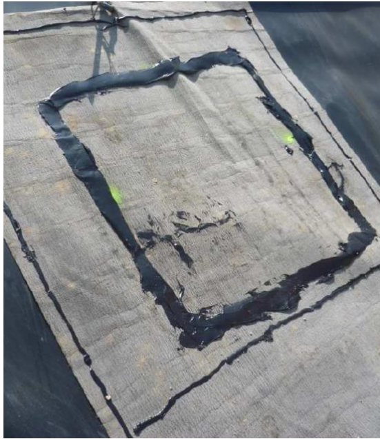
Figura2: Geosynthetic cloth ready to be place
