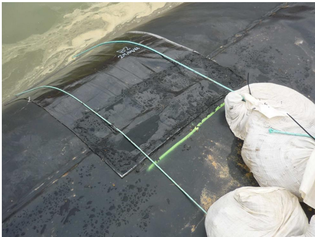
Figura5: Final result of a repaired defect
