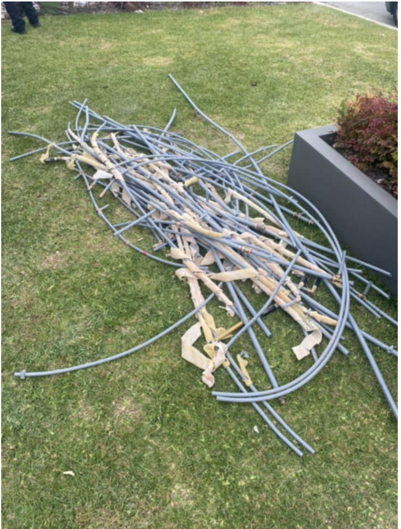
📷 Defective polybutylene plumbing pipes have been stripped out of hundreds of new homes in WA due to water leaks and bursts that have caused huge damage. Credit: Unknown/Supplied
