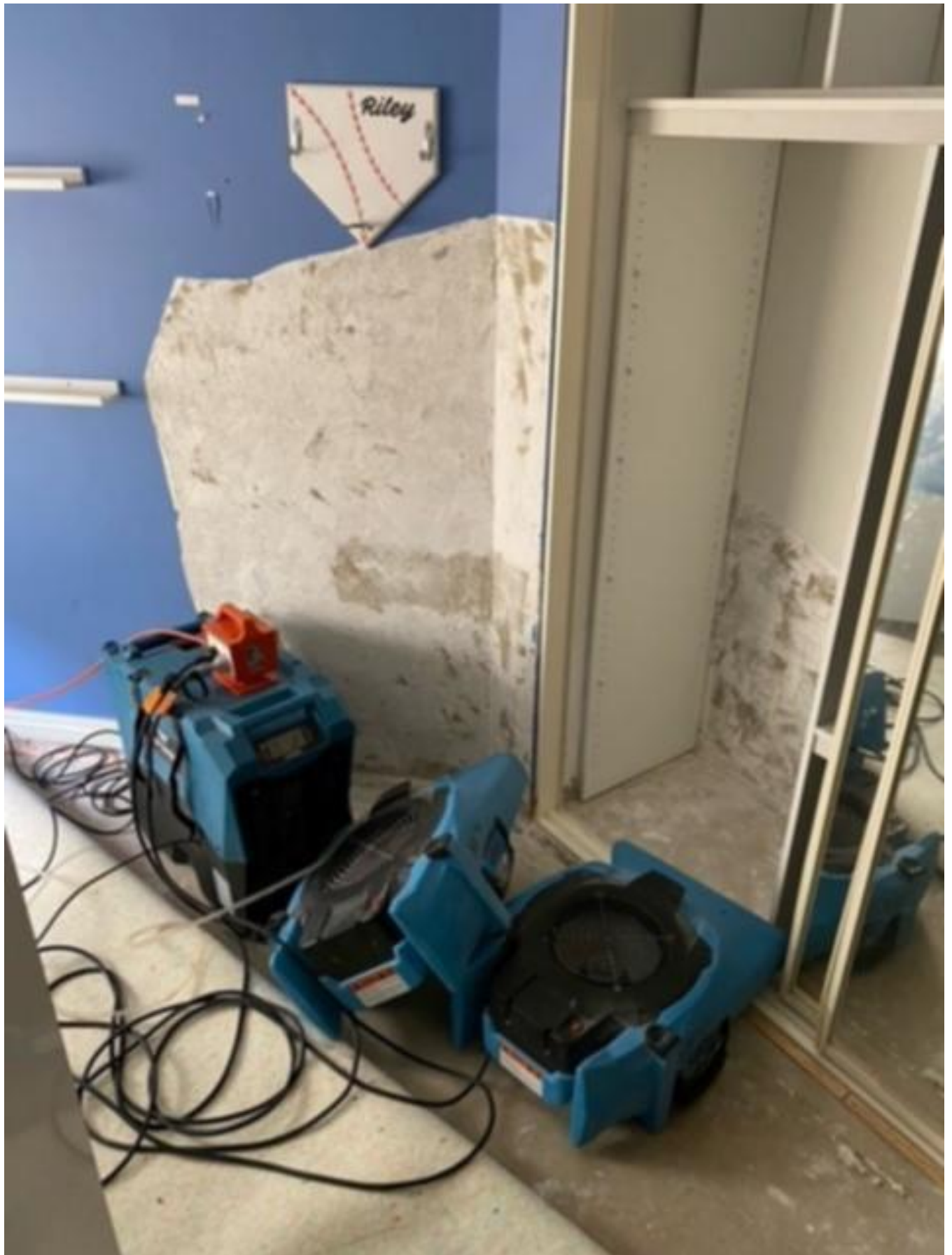
📷 Dehumidifiers in action in the waterlogged Jane Brook home of Damon Connaughton. Credit: Supplied
