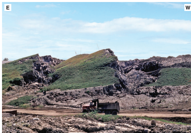
Fig. 8. (Color) Close-up view of Crossroads Landfill failure showing intact waste blocks and scarps caused by retrogressive foundation failure. (Reproduced from Luetlich et al. 2015, with permission of University of Maine)
