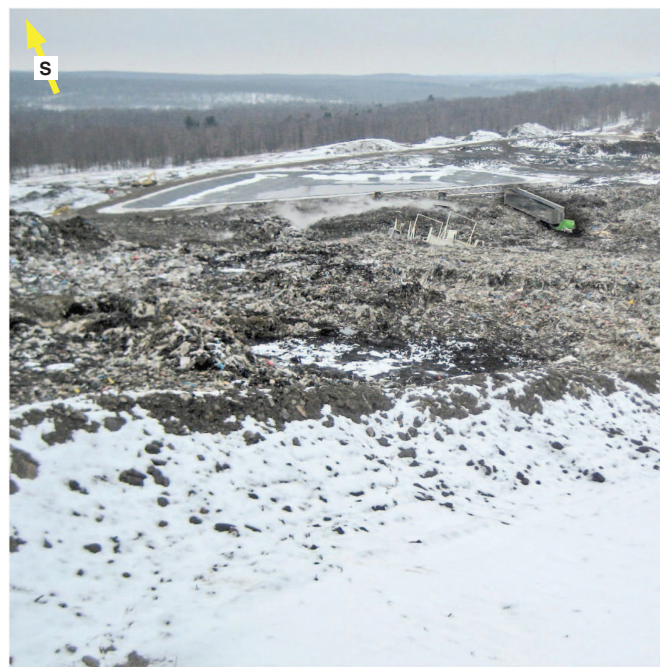
Fig. 23. (Color) Postfailure condition of confidential northeast US MSW landfill Cell 10B/11A, looking south; green truck cab in upper right portion of photo provides sense of scale (photo from project files, taken March 20, 2017). (Image by David J. Bonnett, reproduced with permission from Geosyntec Consultants, Inc.)
