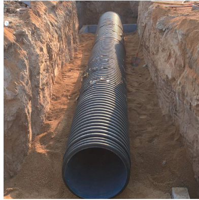
Fig. 2. Example of a High-Density Polyethylene Pipe [1]
