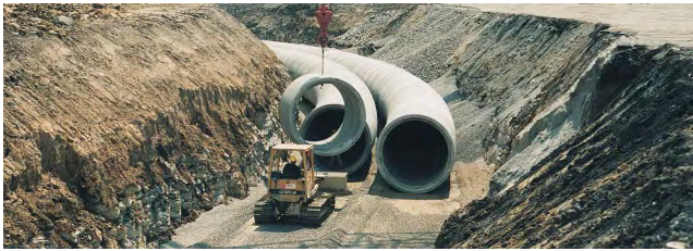
Fig. 1. Example of a Reinforced Concrete Pipe [1]
