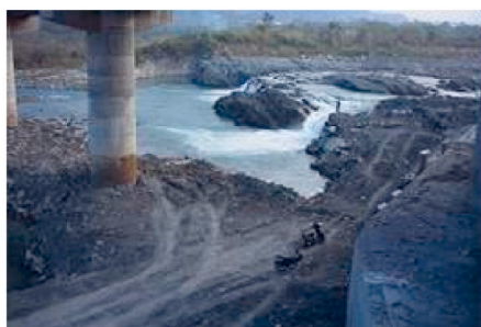
(a) Newly constructed bridge
