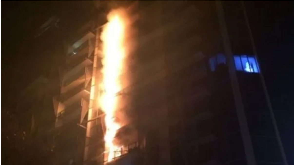
The 2014 cladding fire at Dockland's Lacrosse tower. MFB
