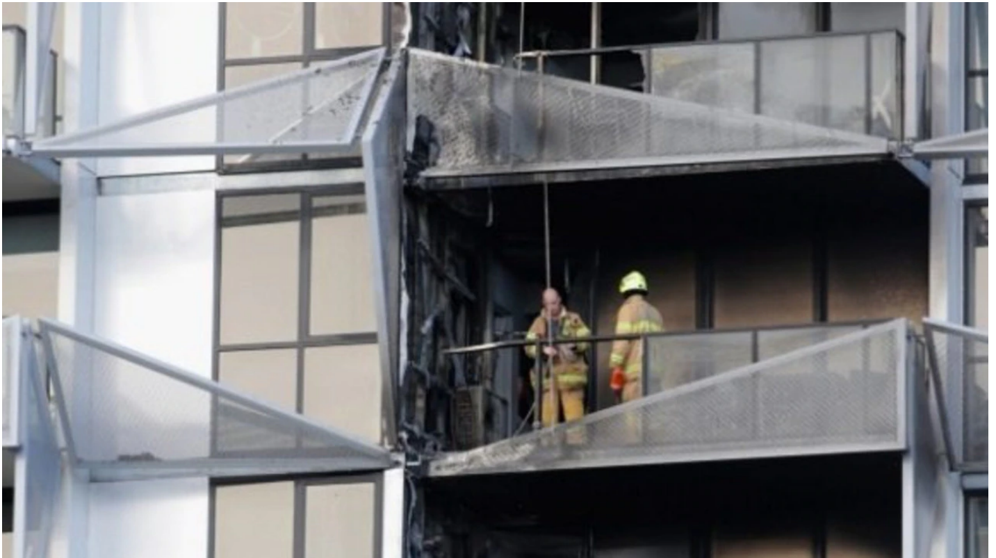
Firefighters check the Lacrosse building in the Docklands after a blaze spread quickly through the cladding in 2014.
