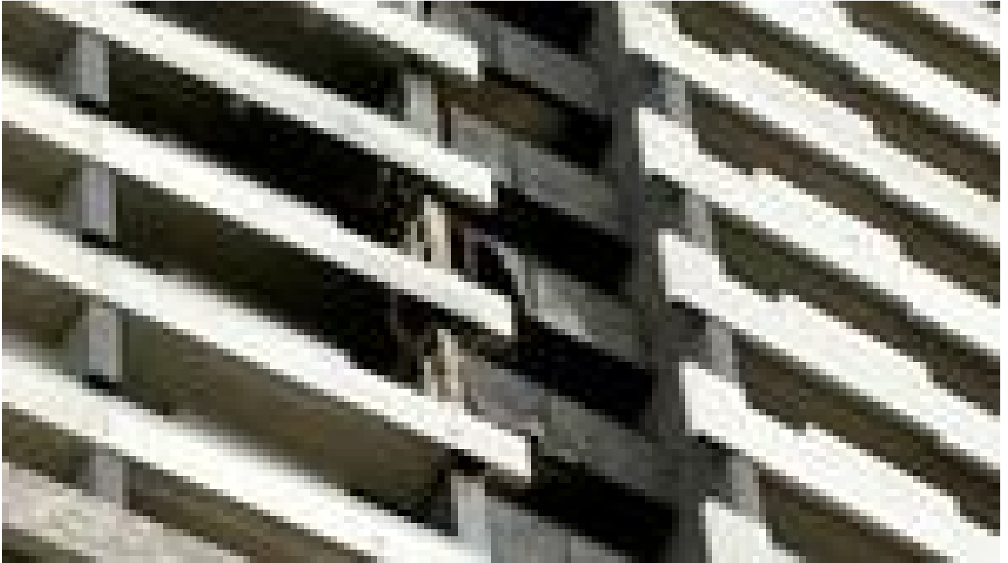
The Neo200 building in Melbourne, which had a fire fuelled by aluminium cladding in 2019. Picture: Stuart McEvoy
