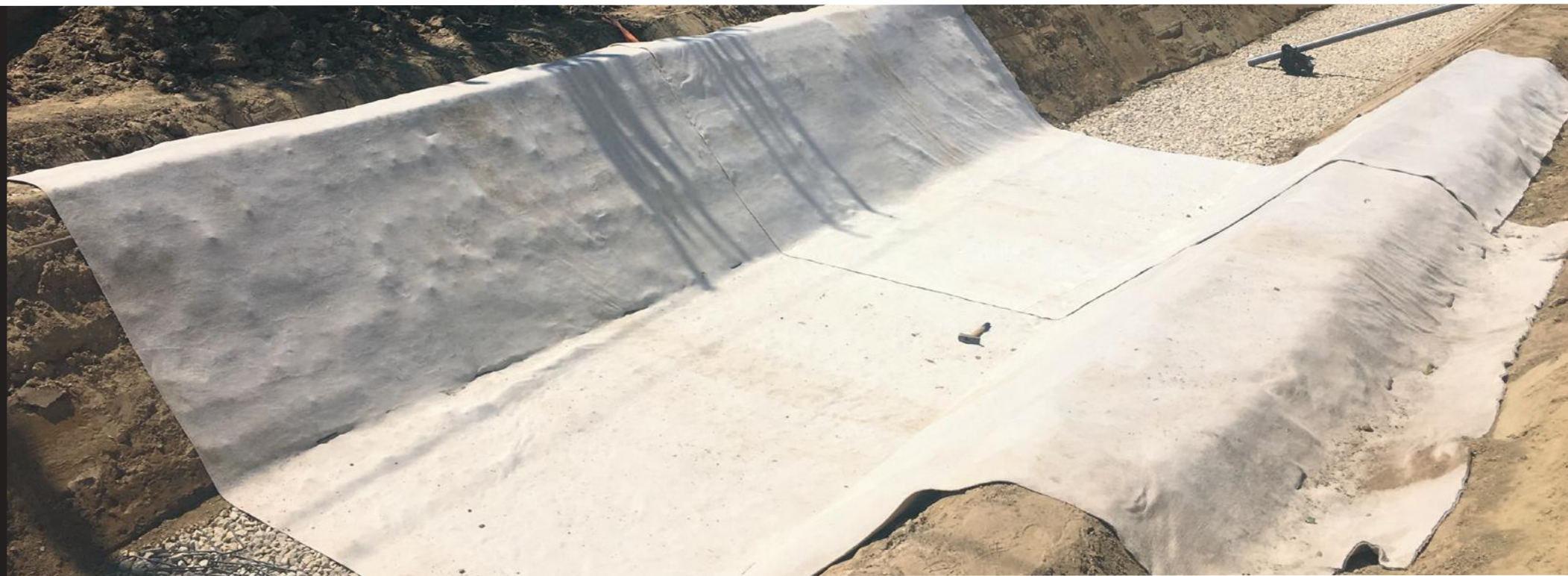
CANAL AND DITCH LINING
