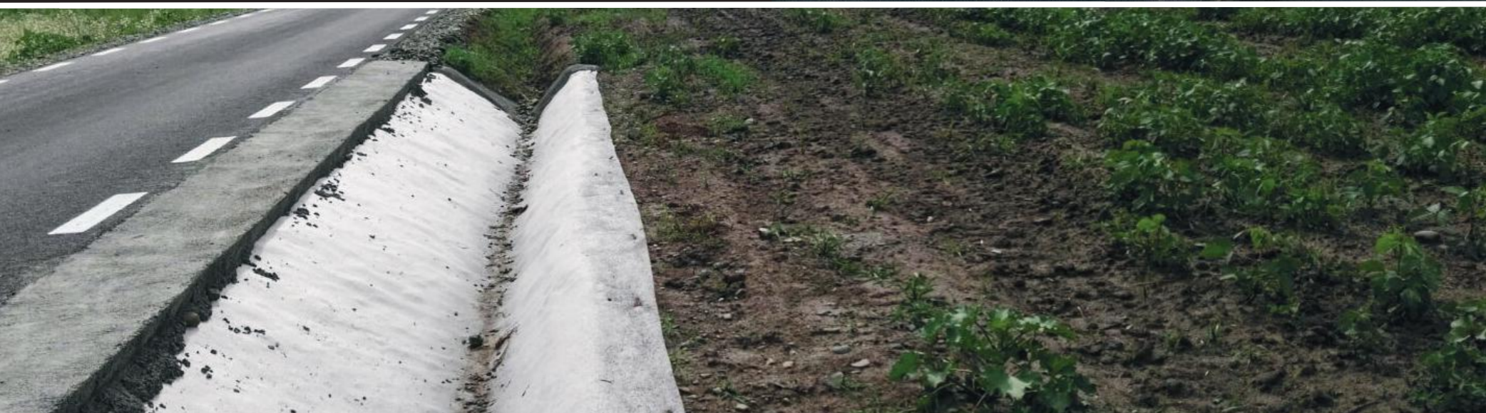
ROAD AND RAILWAY DITCHES LINING
