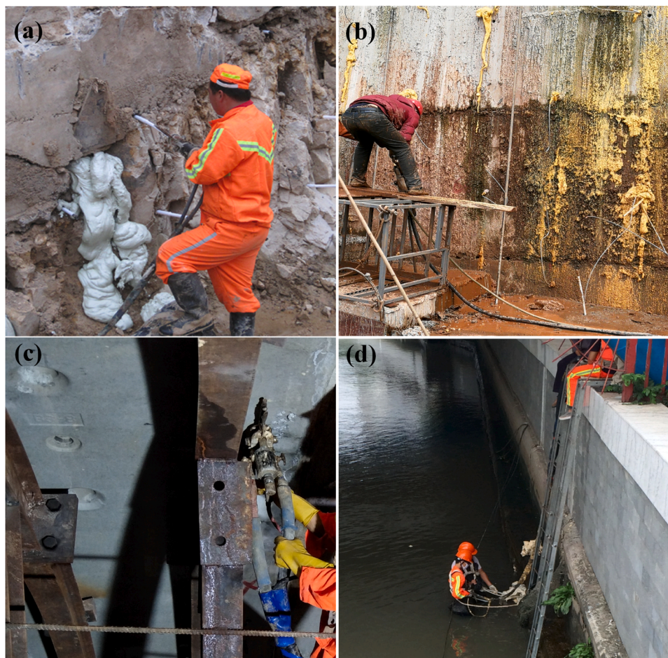
Fig. 1. Application cases of polyurethane grouting materials in China for seepage prevention: (a) a dam; (b) a landfill dam; (c) a shield tunnel; (d) a levee.
