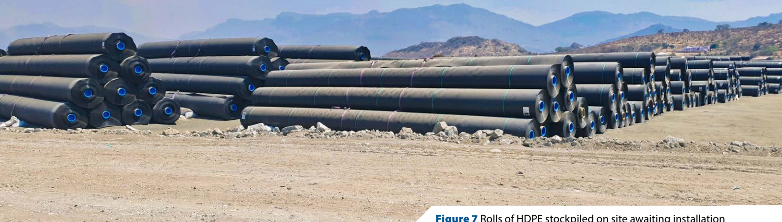
Figure 7 Rolls of HDPE stockpiled on site awaiting installation
