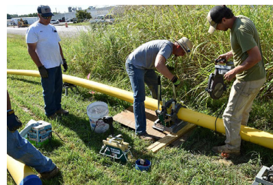
A crew works on an ESPD project in Henderson, Kentucky.
