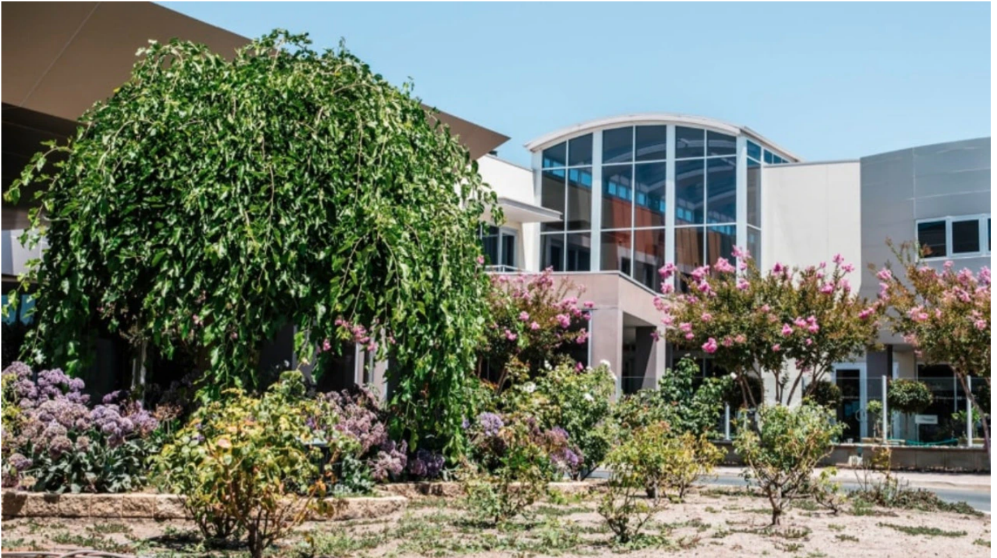
The nursing home appealed a committee notice calling for $250,000 worth of new cladding. Picture: The Society of Saint Hilarion Aged Care / Facebook
