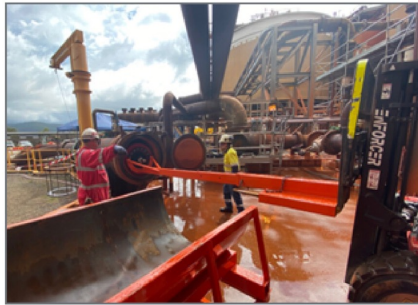
Figure 2: Launcher location during launch of gauging bidi
