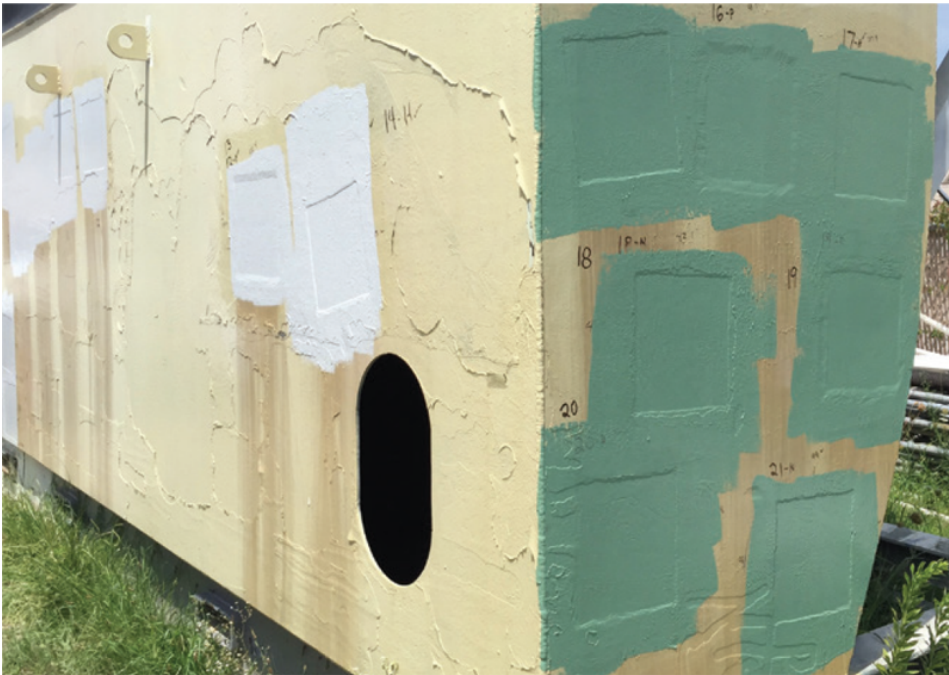
Fig. 4: Mock tank after repair primer.
