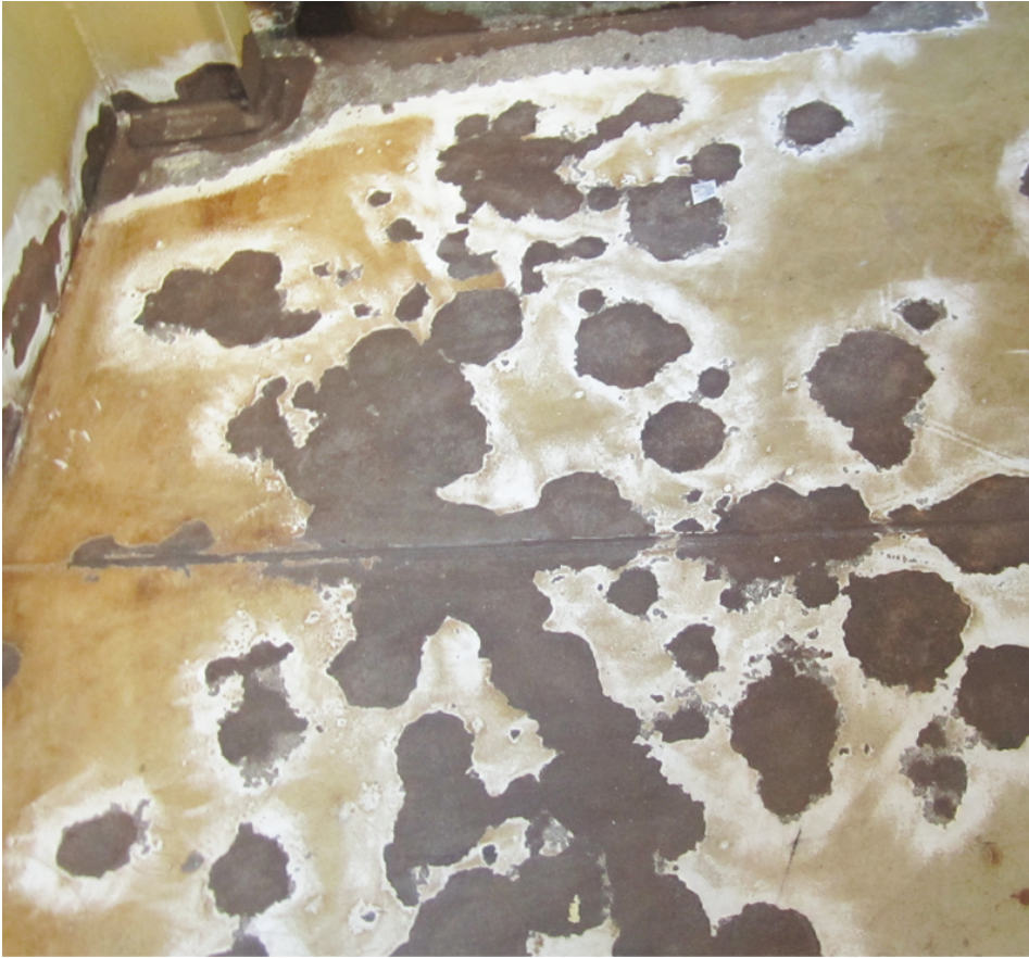
Fig. 1: Feathered intact legacy coating in preparation for maintenance painting. Figures courtesy of the authors.
