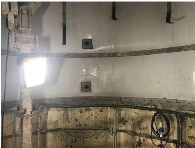
Figure 18.34 PVC composite geomembrane taut to the inner concrete lining
