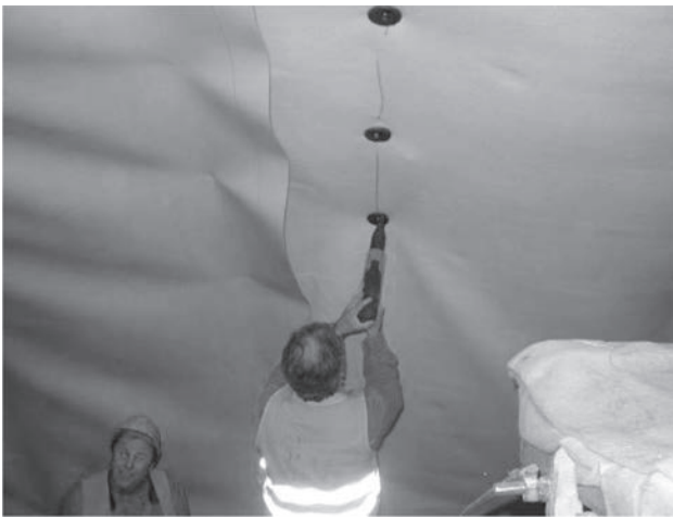
Figure 18.20 Geomembrane heat welded to the roundels
