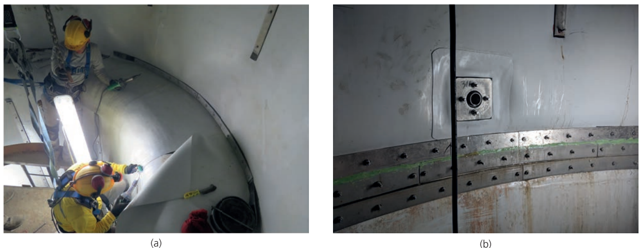
Figure 18.35 Watertight perimeter seals at (a) the connection surge shaft/pressure shaft and (b) the bottom of a compartment
