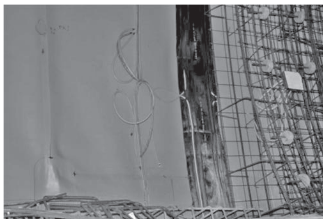
Figure 18.24 Post-grouting arrangement at a waterstop
