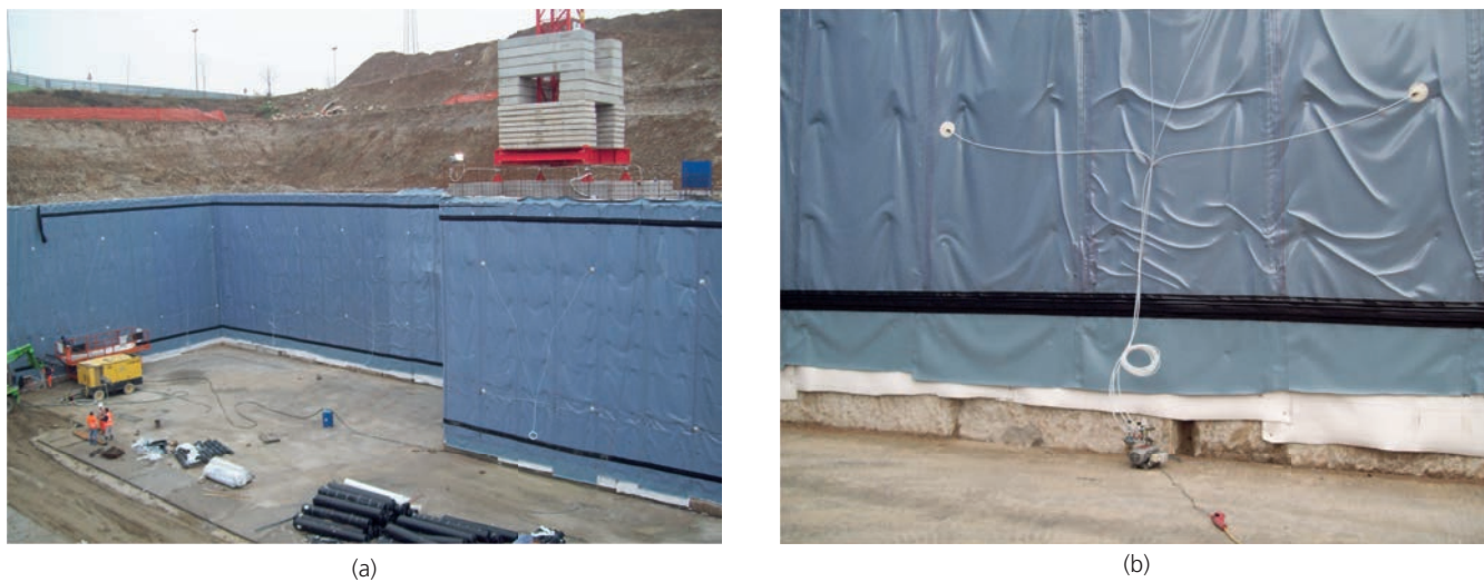
Figure 18.32 Conditions of (a, b) the substrate dictate the selection of (c) the support layer. In this case, possible further opening of cracks required a geocomposite formed by a geogrid with a high bearing resistance and a high modulus, laminated at manufacturing to an anti-puncture geotextile
