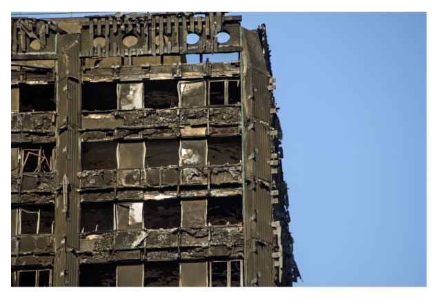
In recent years, the fire risks associated with aluminium composite panel (ACP) cladding have become a pressing concern in the construction industry. While various testing methodologies exist, serious shortcomings in the way cladding materials are analyzed and evaluated continue to put public safety at risk.
