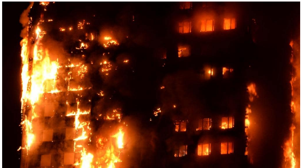
Clad in disaster: Flames engulf the 27-storey Grenfell Tower in London on June 12, 2017. The building had combustible panels with the PE material in it.
