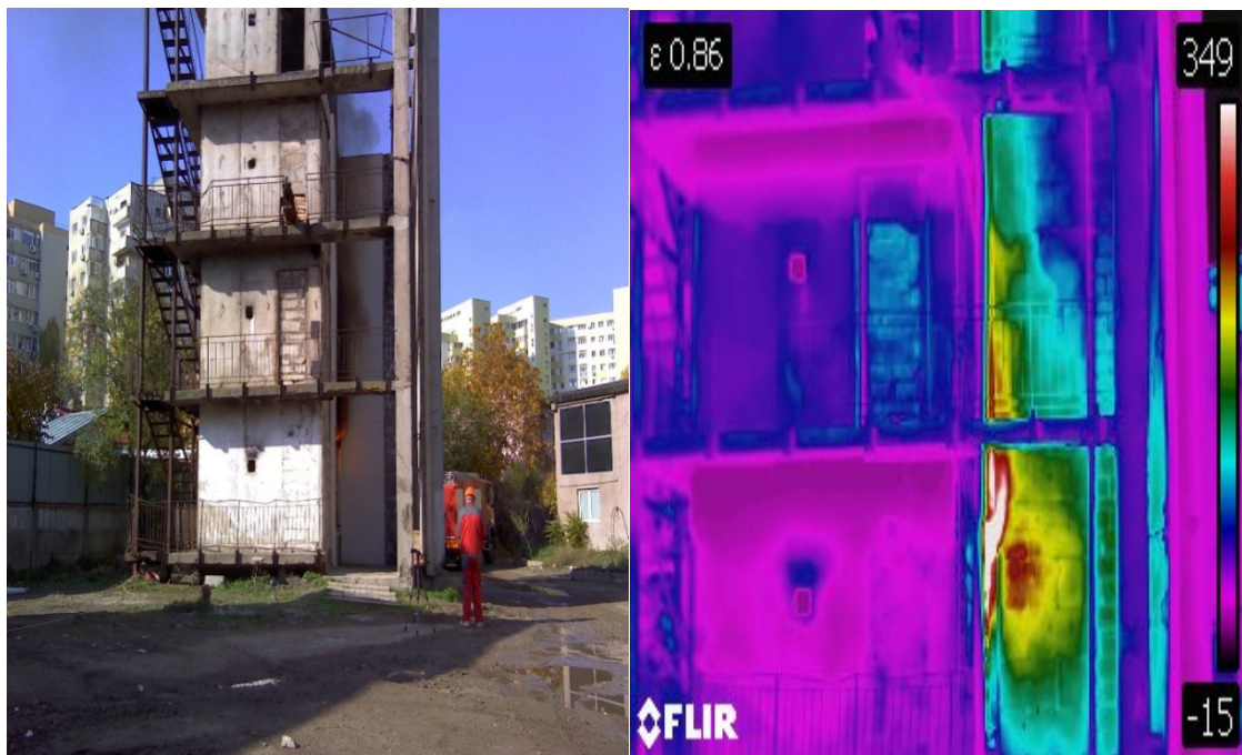
Figure 5. Images (photo and thermal) during the development of the compartment fire
