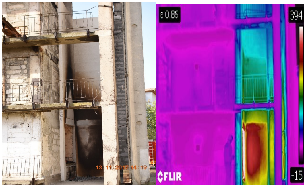
Figure 7. Images (photo and thermal) at the end of the test
