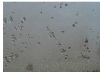
Pitting after cleaning and abrasive blasting – the surface alternates between pits and smooth regular areas
