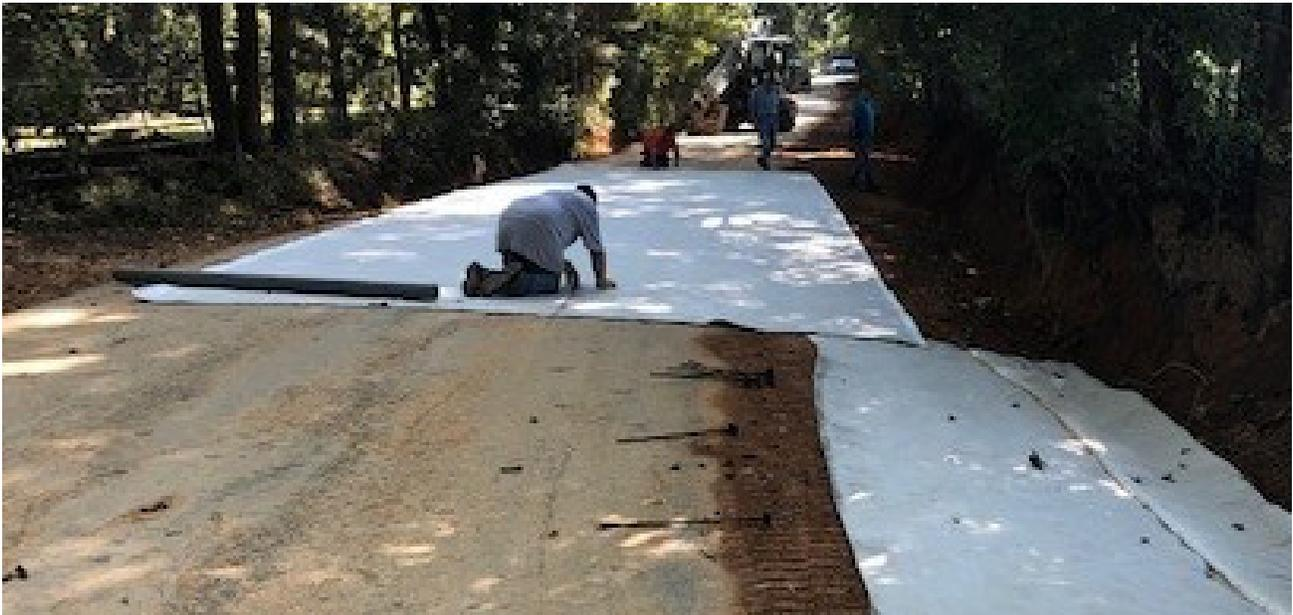
The RCR® material was unrolled and cut to size by using a utility knife. After the RCR® material was cut to size, it was slid into position by hand and pinned into place. This was done by driving rebar pins with plates welded to the top into the bank.
