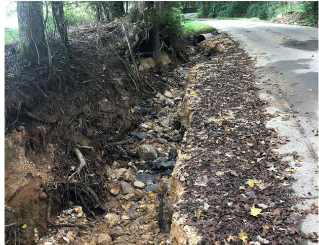
For many years the Department of Public Works would have to go in and build-up this 850' long ditch after any heavy rains. This of course was very costly due to several reasons including labor, machinery, material and of course having the road shut down. Because of this road being used by school buses, as well as local traffic, it had to be taken care of right away every time there was a heavy rain.
