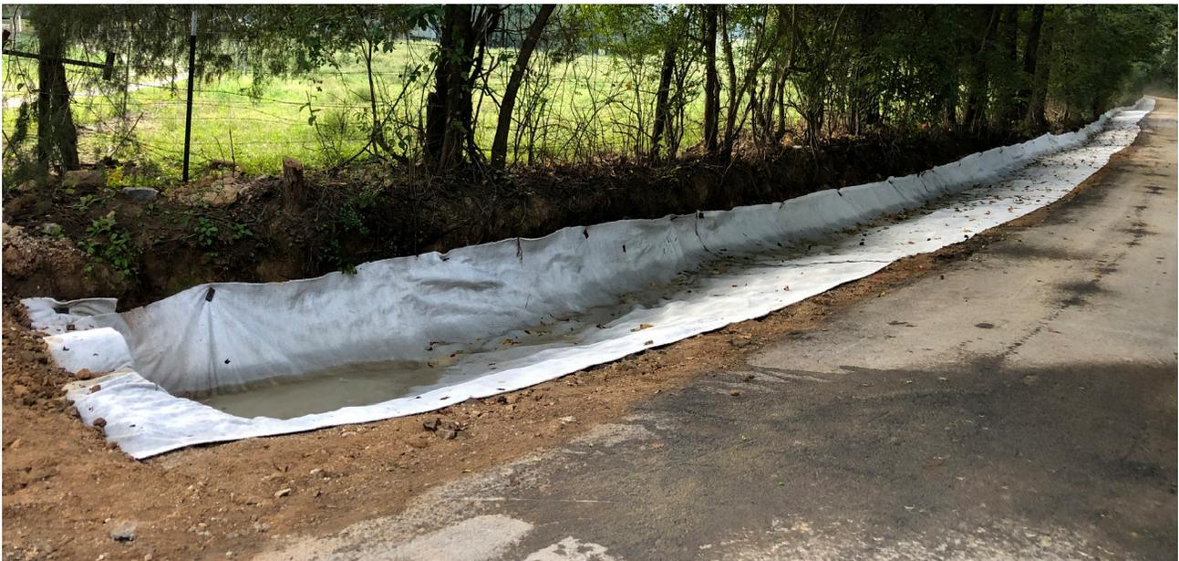
The total install of approximately 850 FT. of ditch was lined in 1 day. That even included the customizing of the RCR® to the existing culverts.
