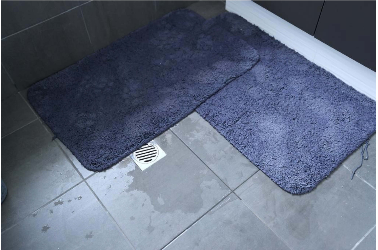
Thousands of WA homeowners are impacted by the defective Iplex pipe saga. Credit: Daniel Wilkins/ The West Australian
