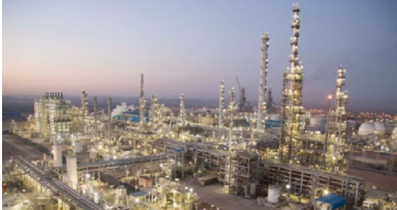
Ethylene plant in Egypt.
