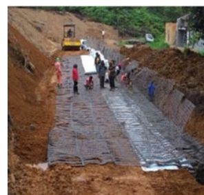
Fig. 3 Geosynthetic reinforced soil structures for slope stabilization and landslide rehabilitation in Asia (from Rimoldi et al. 2021): a reinforced soil structure along the river Myittha in Myanmar, as a remedial work of an existing collapsed concrete masonry wall, b installation of gravel layer wrapped with nonwoven geotextile as drainage material, c rainwater runoff triggered a slope collapse, and d installation of geosynthetic reinforcements and view of the completed slope remediation
