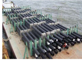
Figure 4—New HDPE Line during installation activities
