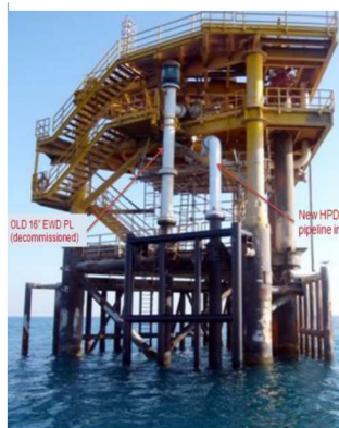
Figure 5—New HDPE pipeline in service (Right)
