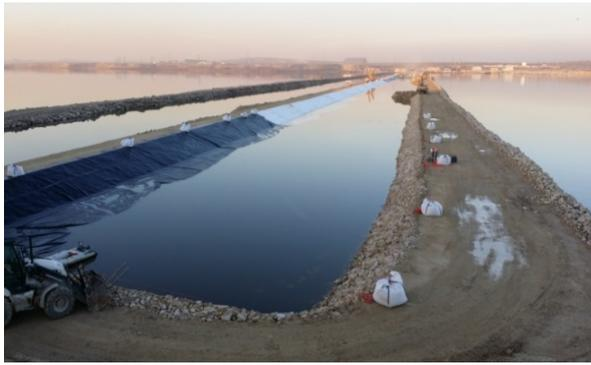
Figure 15. Road Dam Geomembrane Installation (Genap, 2015)
