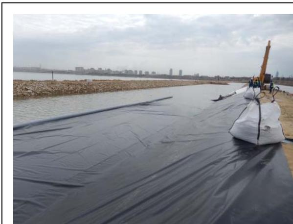
Figure 10. Floating geomembranes panels before submerging under water (Witteveen+Bos supervision staff, 2015)
