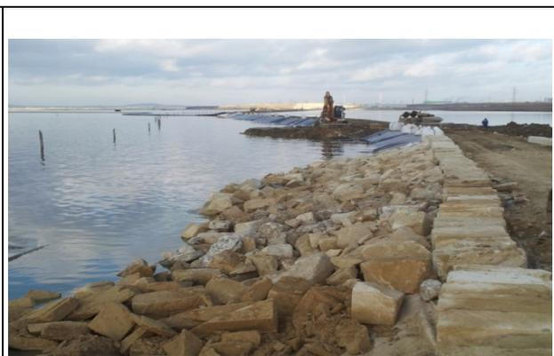
Figure 14. North Dam Geomembrane Installation (Genap, 2015)
