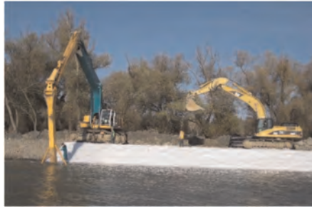
Figure 7. Installation of geocomposite sandmattress as filter layer below a stone revetment.
