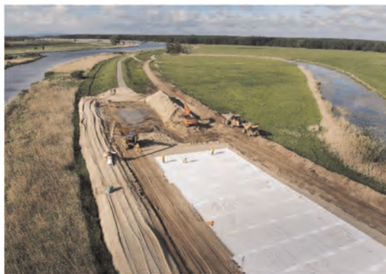
Figure 16. Installation of high strength geogrids as basal reinforcement below the flood defence at the Oder dike, Germany.
