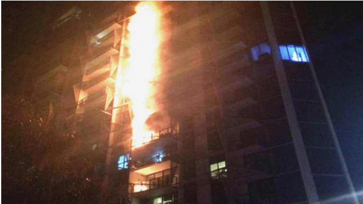
The Lacrosse tower fire in Melbourne's Docklands in 2014. Credit: Metropolitan Fire Brigade/Metropolitan Fire Brigade
