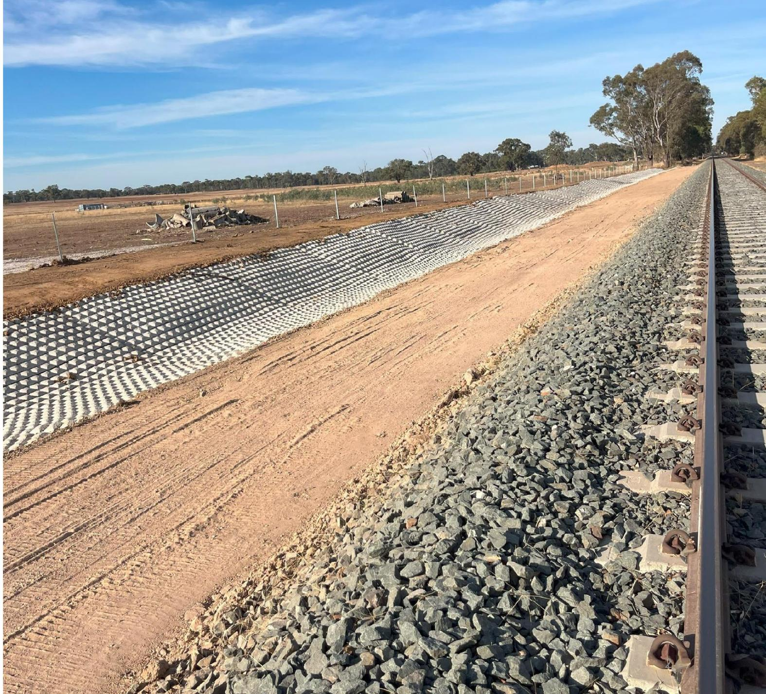
***“Earthlok delivered 7m x 5m wide rolls and the 220m long drain was completed in just days”***
