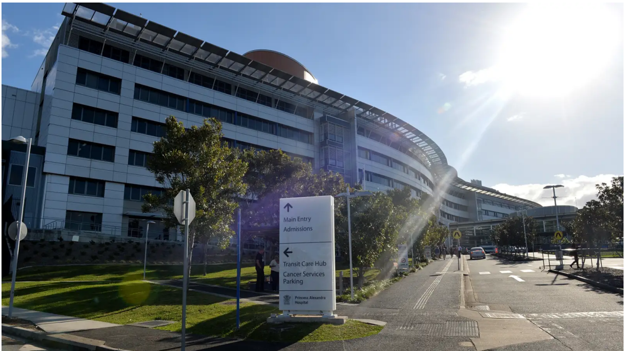
Cladding was removed from the Princess Alexandra Hospital. BRADLEY KANARIS/FAIRFAX MEDIA
