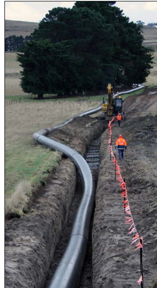
Midland Irrigation project Tasmania
