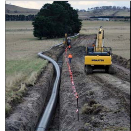
Midland Irrigation project Tasmania
