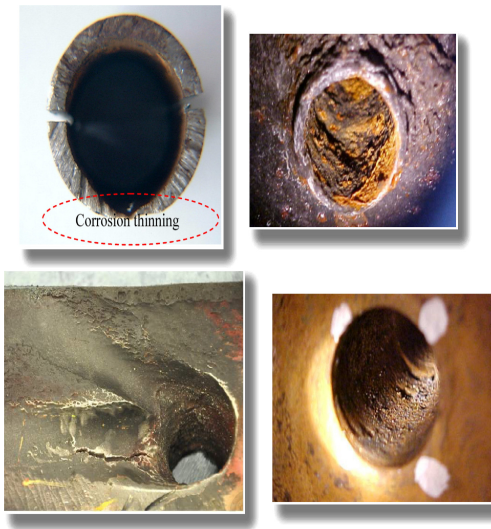
Fig. 10 Some failure parts caused by ammonium bisulfide ( \text{NH}_4\text{HS} ) [65,70].
