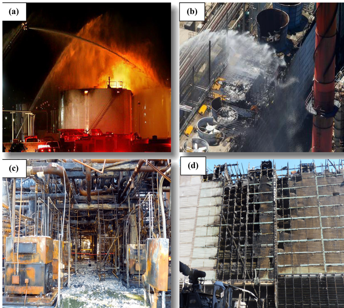
Fig. 1 Examples of some refinery's accidents caused by corrosion failure. (a) Golden Eagle Refinery, (b) Richmond Refinery, (c) and (d) Chevron Refinery.
