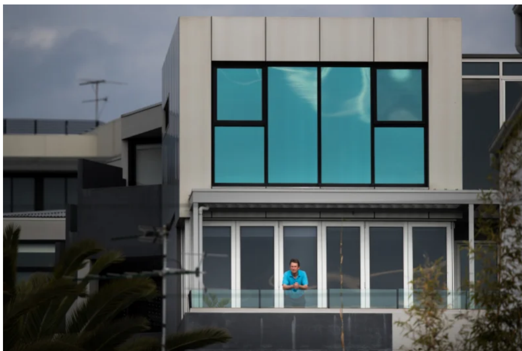
Neill Fitzpatrick on the balcony of his Port Melbourne apartment. Rates on his property have not fallen, despite cladding needing to be rectified on it. JASON SOUTH
