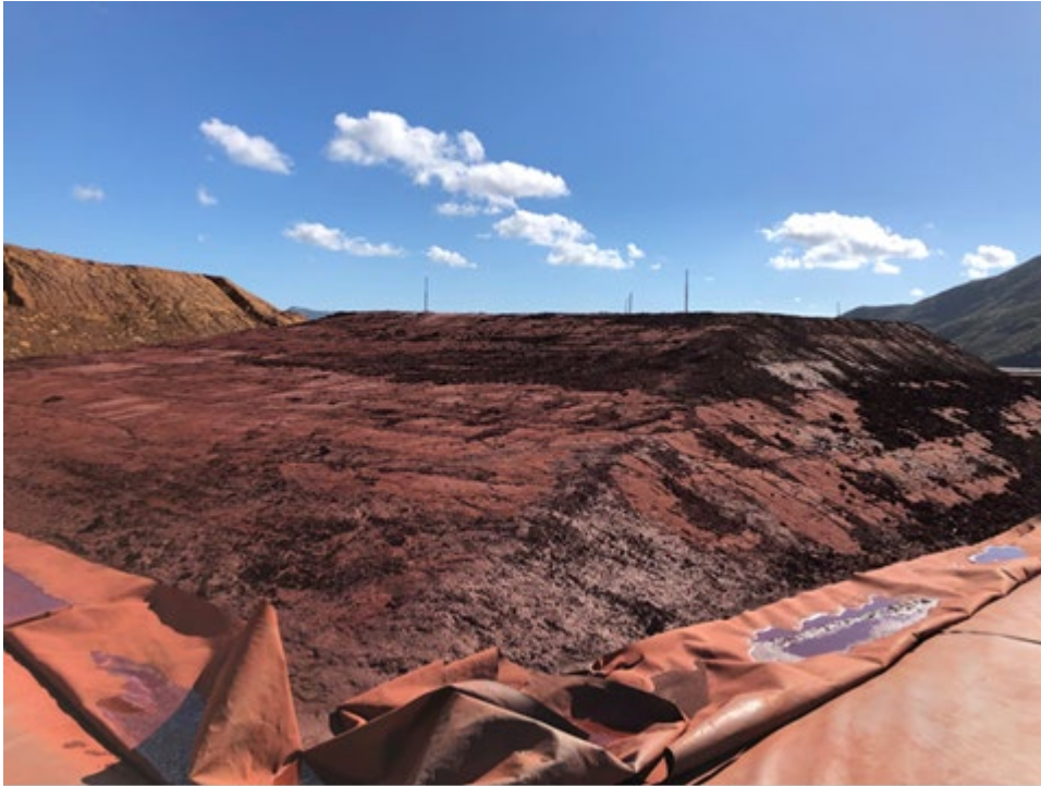
Figure 5: Condition of Compacted Residue Slope Batters approximately One Year after Construction
