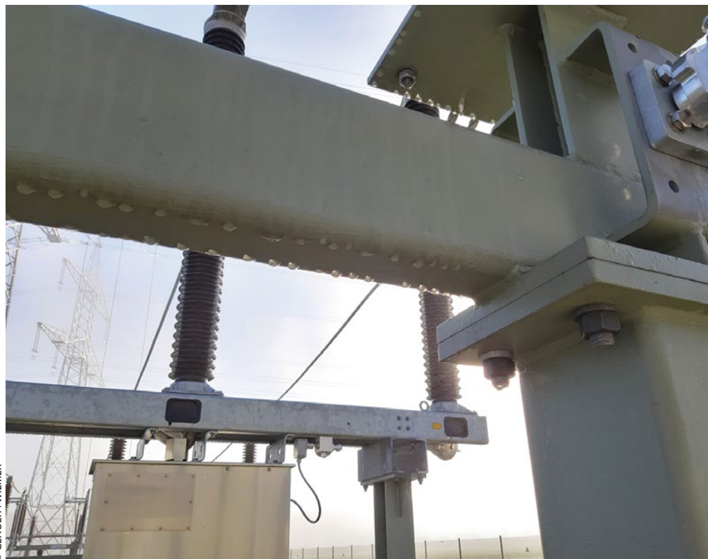
Fog and dew – usually unfavorable conditions for coating work.
