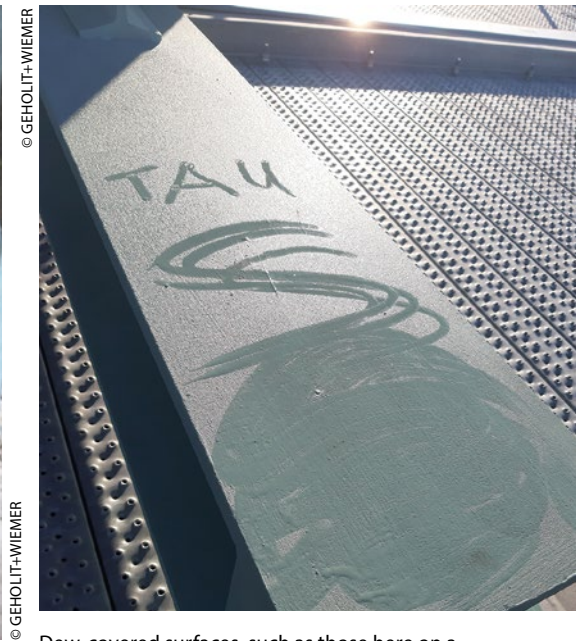
Dew-covered surfaces, such as those here on a transformer substation, can be coated directly.
