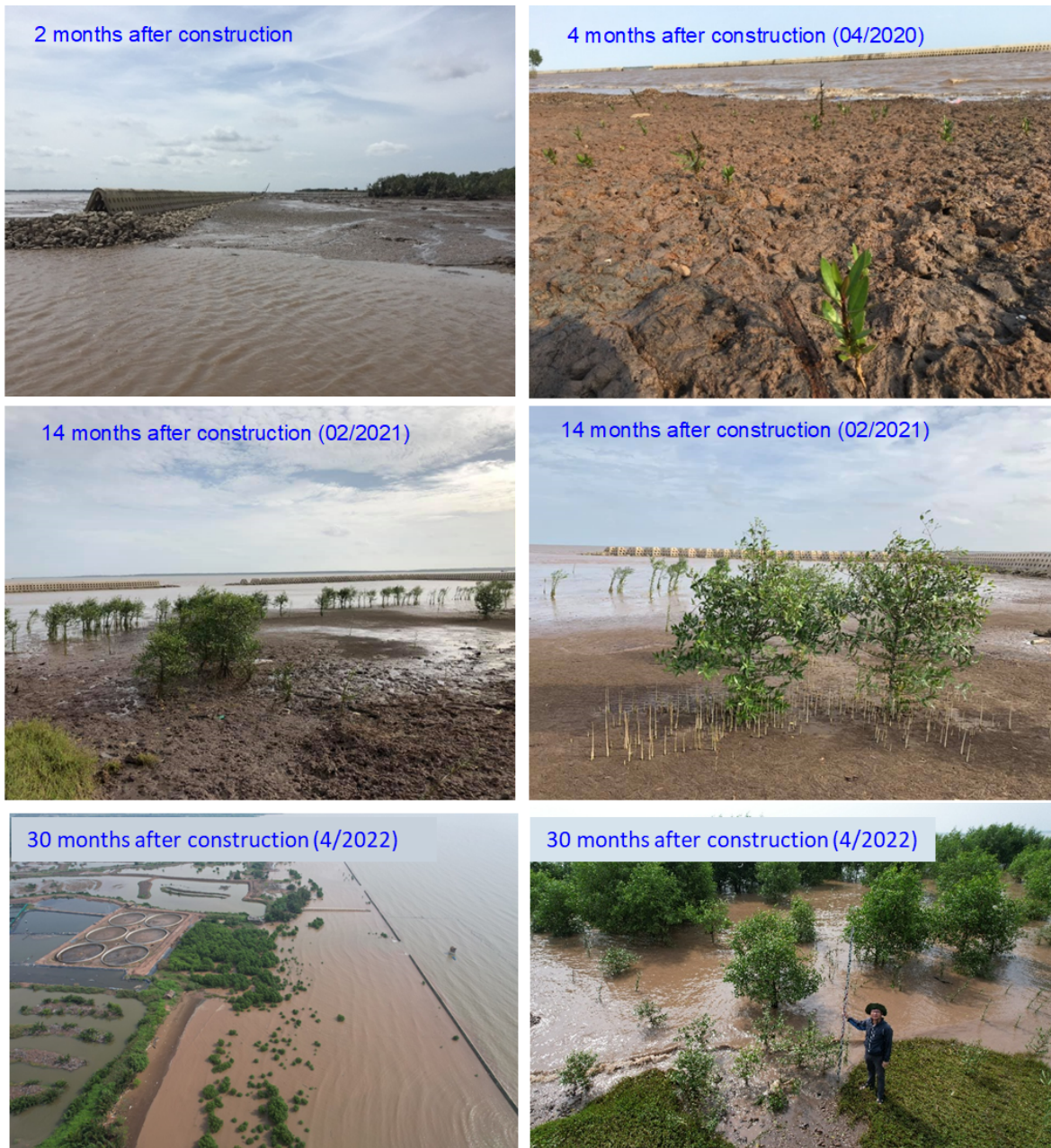
Figure 15. The sedimentation and the restoration of mangrove apple ( Sonneratia caseolaris ) behind the dyke (right) at Con Cong coast – Tien Giang (Source: SIWRR, 2021)
