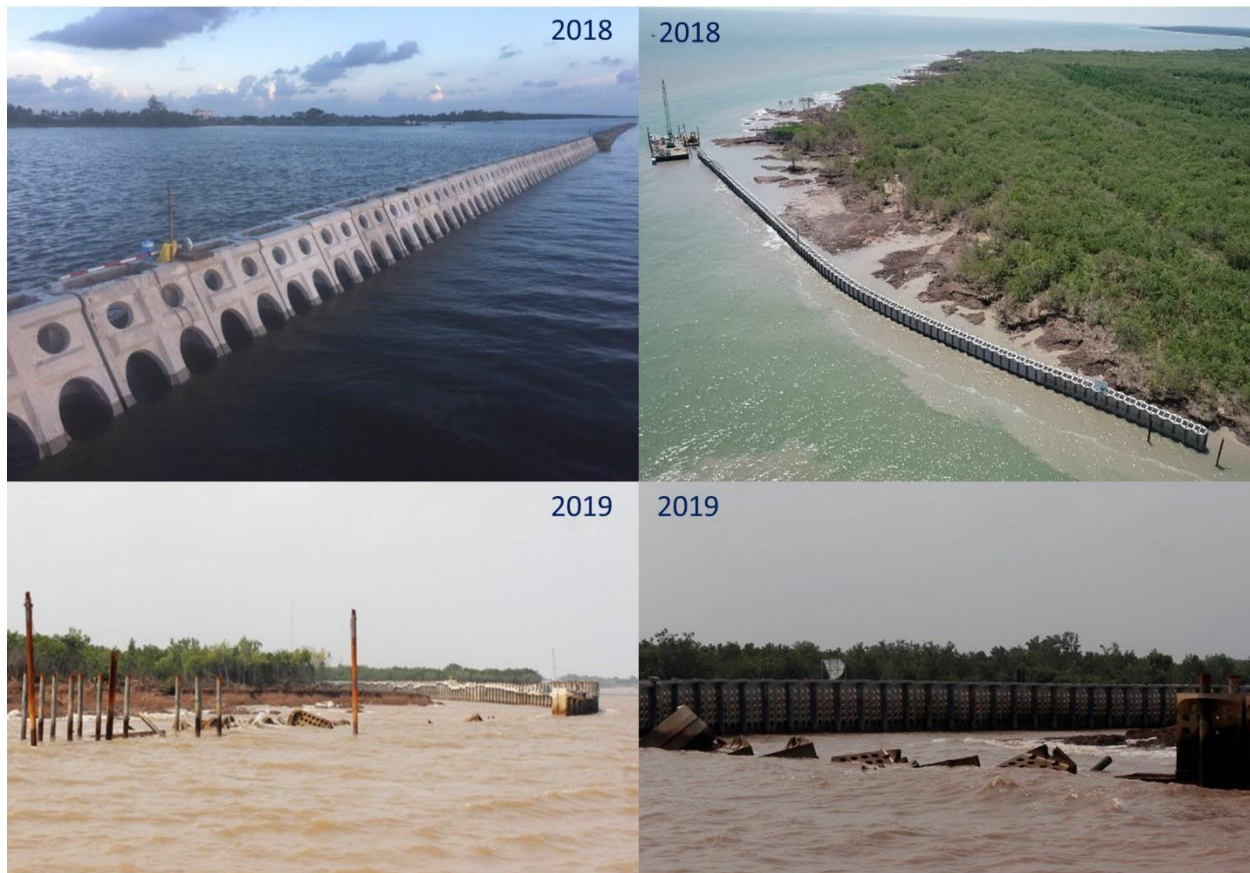
Figure 12. The Busadco’s hollow breakwater was constructed in the West (left-top panel) and East Seas, Ca Mau coast (Source: SIWRR, 2020)
