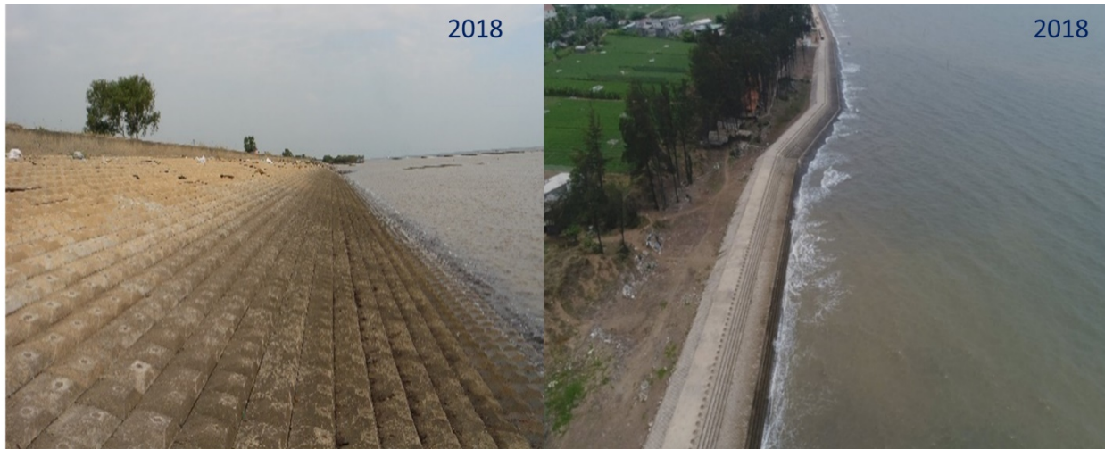
Figure 7. The revetments constructed in Go Cong, Tien Giang and Long Hoa, Tra Vinh, VMD
