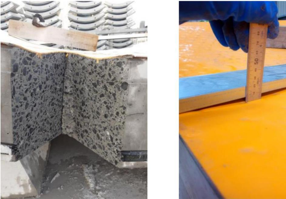
Figure 10. Photo of HDPE lining bulging (photo courtesy of Wilson Tunneling)
