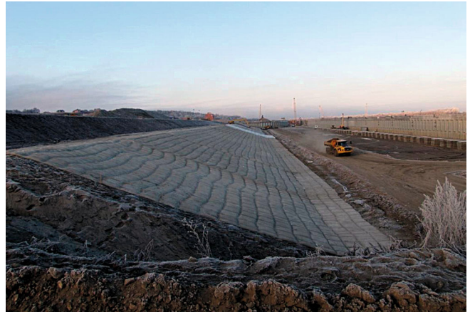
Fig. 15. Reconstruction of the approach channels of the Kuzminsky gateway.
