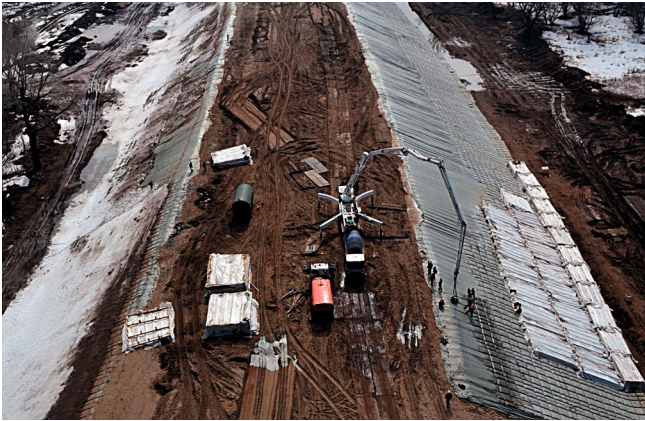
Fig. 14. Bank protection of the approach embankment of the Kirovsky bridge.
