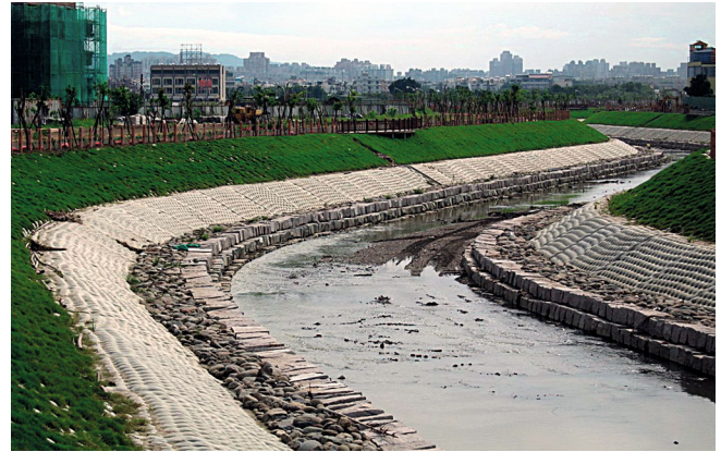
Fig. 13. Combined use of Incomat® Filterpoint and Crib.
