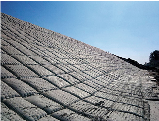
Fig. 12. Fastening of slopes with Incomat® Flex.
