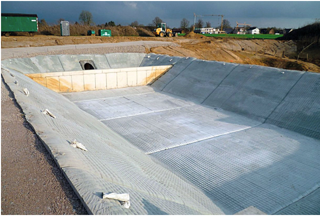
Fig. 11. Waterproofing a pool with Incomat® Standard.
