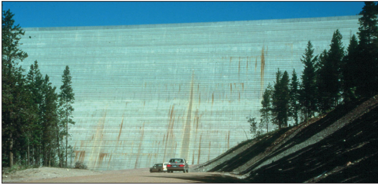
Downstream face of the Upper Stillwater RCC dam.
