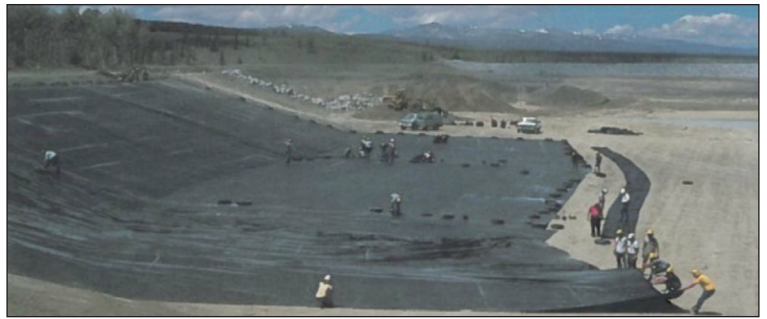
Installation of the geomembrane at Mt Elbert.
