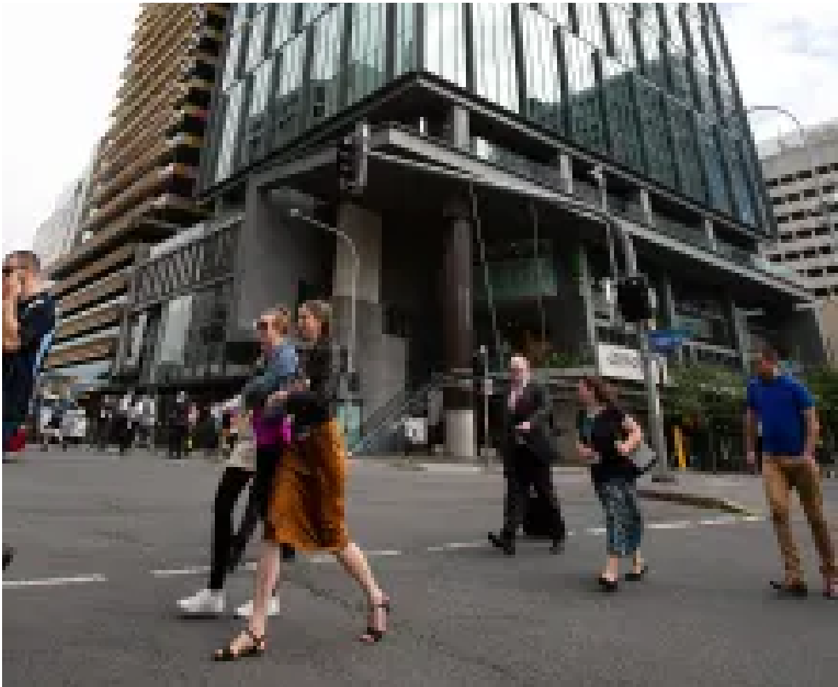
The 34-level 400 George Street tower in Brisbane is tendering to replace cladding that Queensland does not allow, but would be acceptable in NSW and Victoria. Attila Csaszar
