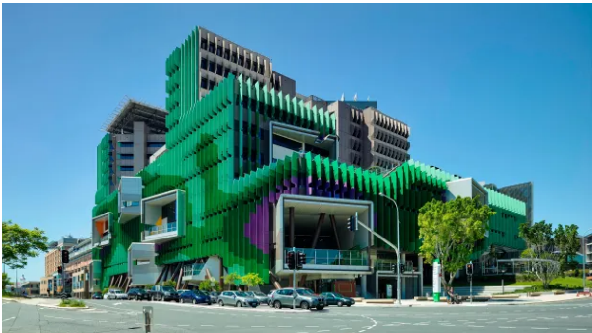
Queensland Children's Hospital is clad in panels with a level of polyethylene content not allowed under state laws. Christopher Frederick Jones
