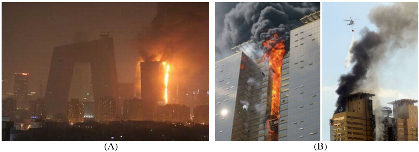
FIGURE 3 (A) Incident at the new CCTV tower on fire 50 and (B) Wooshin Golden Suites, Busan South Korea 51
