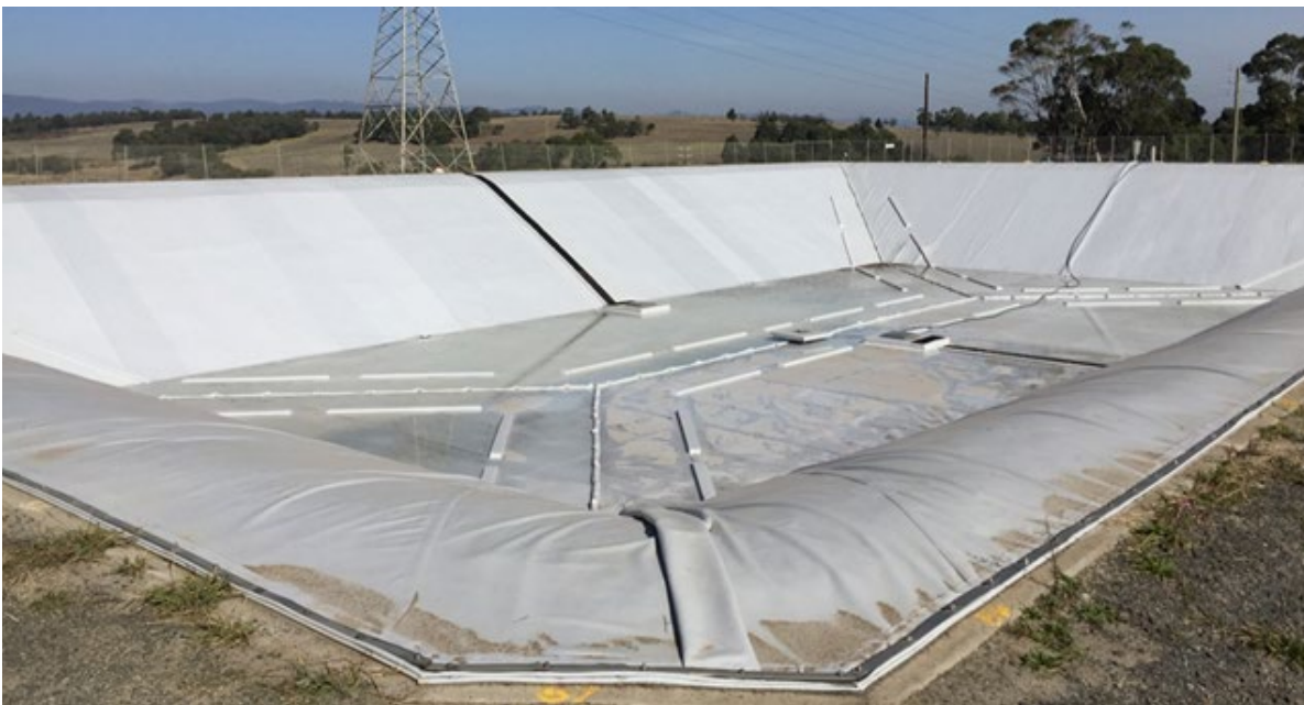
Figure 1: Photograph of grey 60-mil reinforced EIA geomembrane used to create floating cover systems for potable water.
