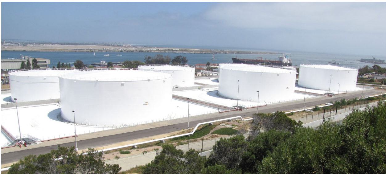
Figure 5: Photograph of white 40 mil unreinforced EIA geomembrane for a secondary containment application without a soil cover.
