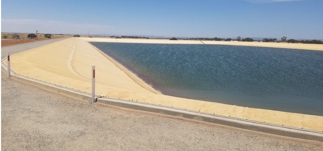
Figure 2: Photograph of tan 60-mil reinforced EIA geomembrane used in a bottom liner system for a water reservoir.
