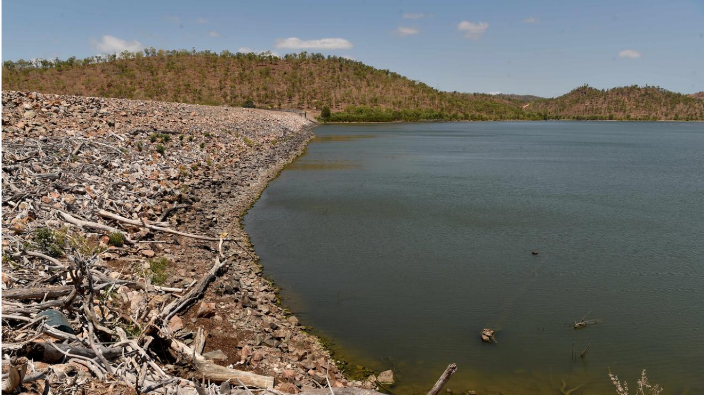
The Ross River Dam. Picture: Evan Morgan
