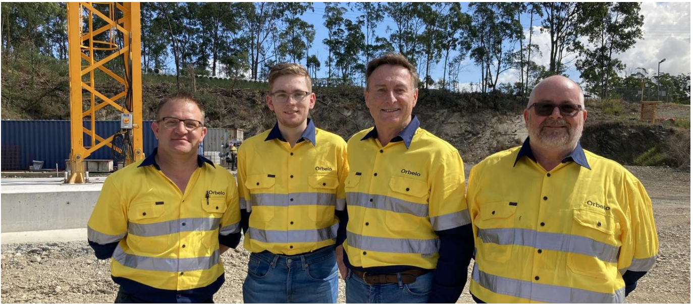
Orbello Edrich Venter, Ben Main, Peter Main and Don Grinstead are part of the team working on the rehabilitation of the tailings dam and mine entrance to the El Dorado gold mine.
