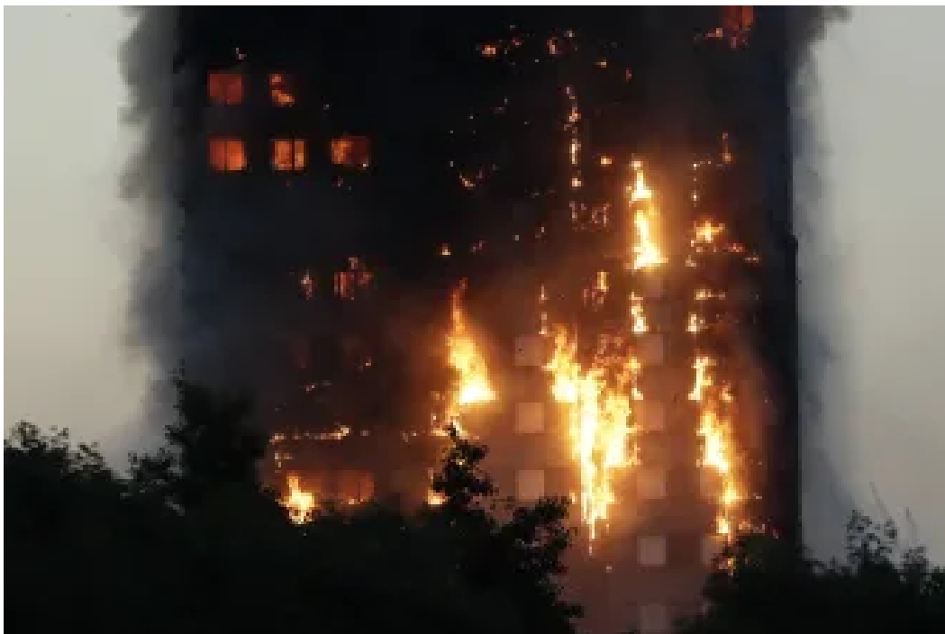
Combustible cladding on London's Grenfell Tower exacerbated a fire that claimed 72 lives in 2017. AP
