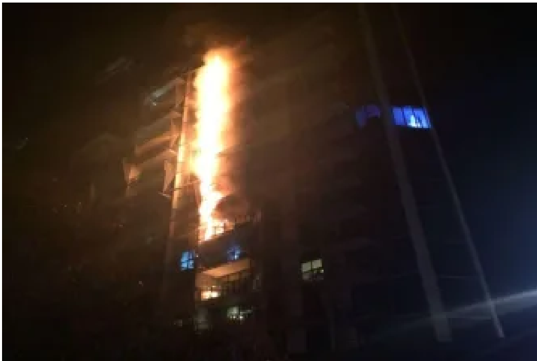
Fire tears up the side of Dockland's Lacrosse building in 2014. The fire prompted a review of flammable cladding on apartments.MFB
