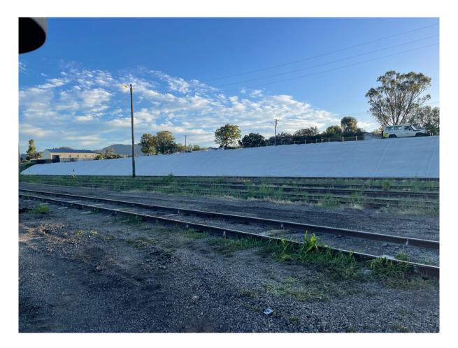
Tiltex 10B GCCM was specified as the ground surface erosion control over the embankments and drains for ARTC's Werris Creek Reconditioning Project. Safety, time management and a durable, low maintenance product were all critical elements of this project's success.
