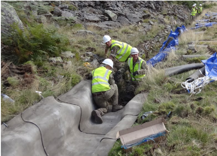
The 75 Engineer Regiment under 4 2 Brigade at work
