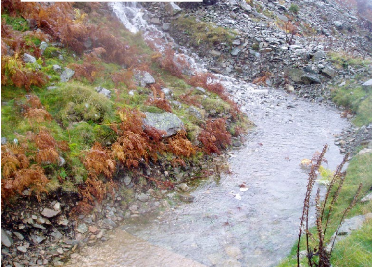
The channel prior to remediation
