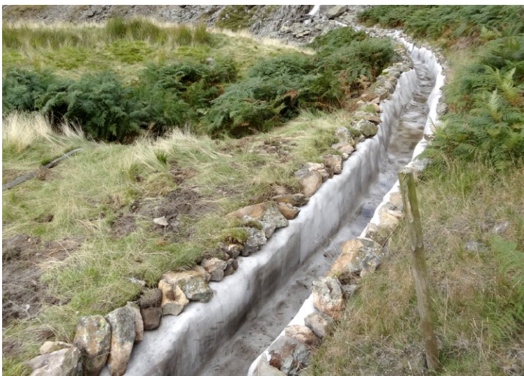
The completed lined channel at Glenridding, Ullswater
