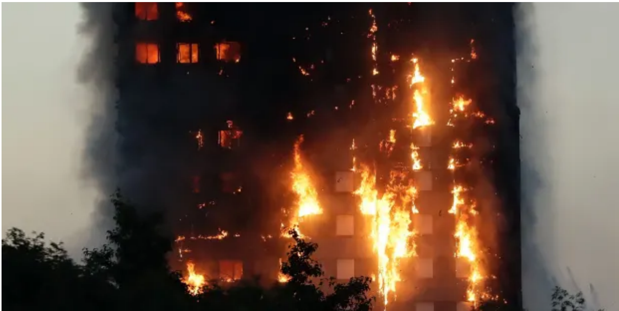
Flames rise from the Grenfell Tower building on fire in London where 72 people died. AP
