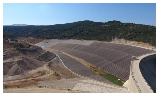
The remarkable height of the dam (70 metres) required the execution of specific product tests by a qualified external laboratory to guarantee the watertightness of the geomembrane under the operating conditions. Siplast's Teranap passed the test successfully, withstanding a pressure of at least 10 bars. Waterproofing test with
