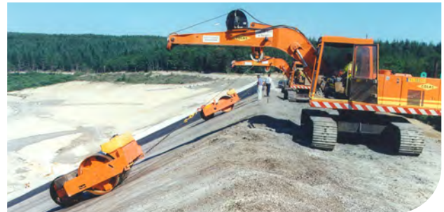
▲ Excavator working along the laying strip, allowing fine leveling of the subgrade before laying the geomembrane
