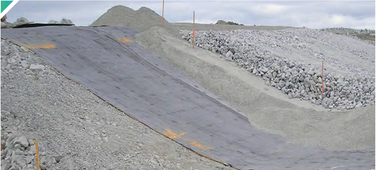
▲ Protective structure of compacted gravel
