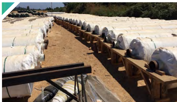
▲ Storage using wooden beams
