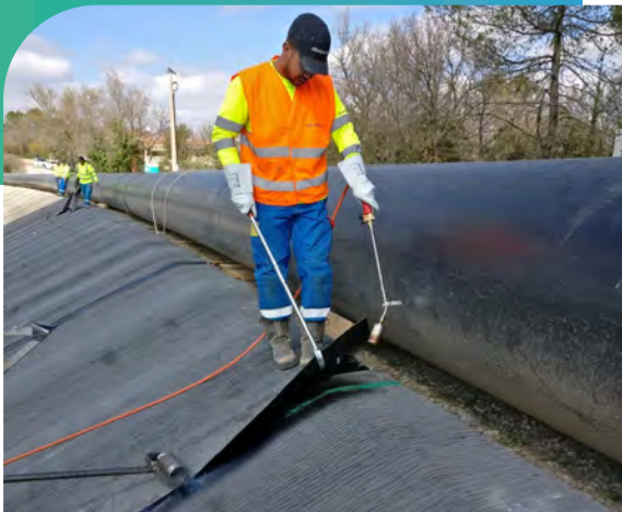
▲ Torch head between the two strips
