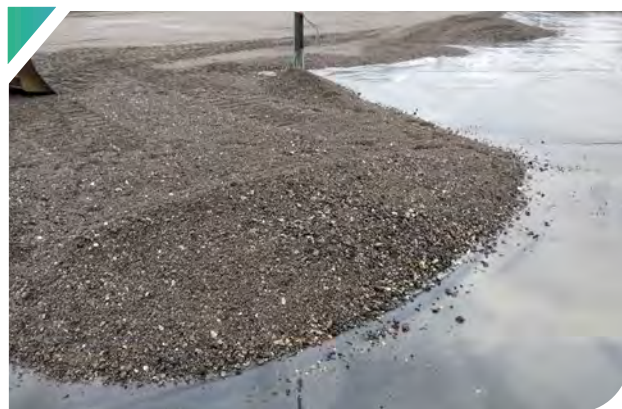
▲ Laying rolled gravel on Coletanche
