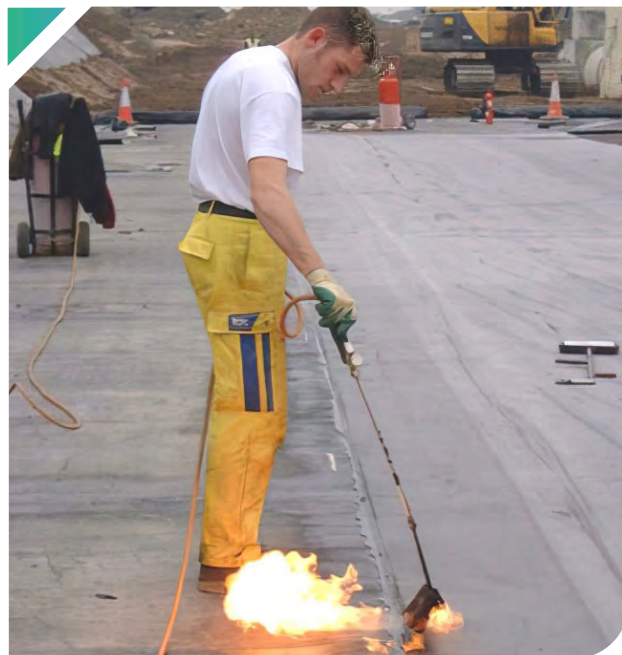
▲ Finishing works with a gas burner and a trowel
