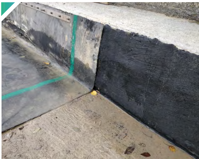
▲ Connection to a concrete block: torching on primed wall and applying mastic
