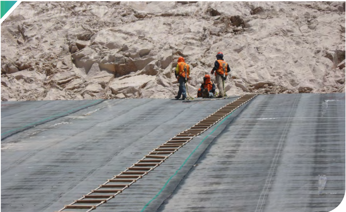
▲ Rope ladders must always be installed on a slope.
