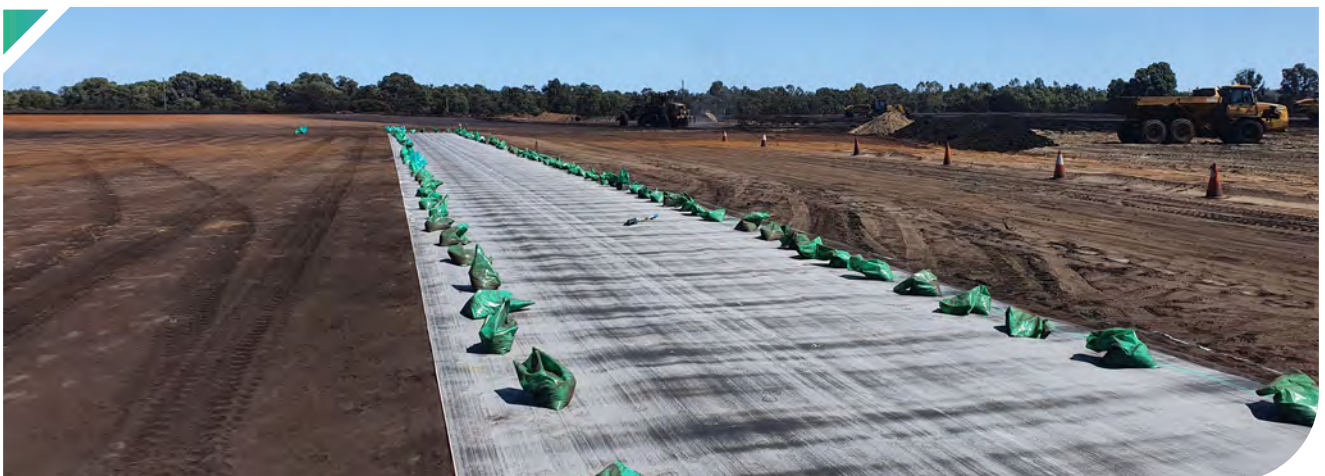
▲ Backfilling materials used as a temporary ballasting
