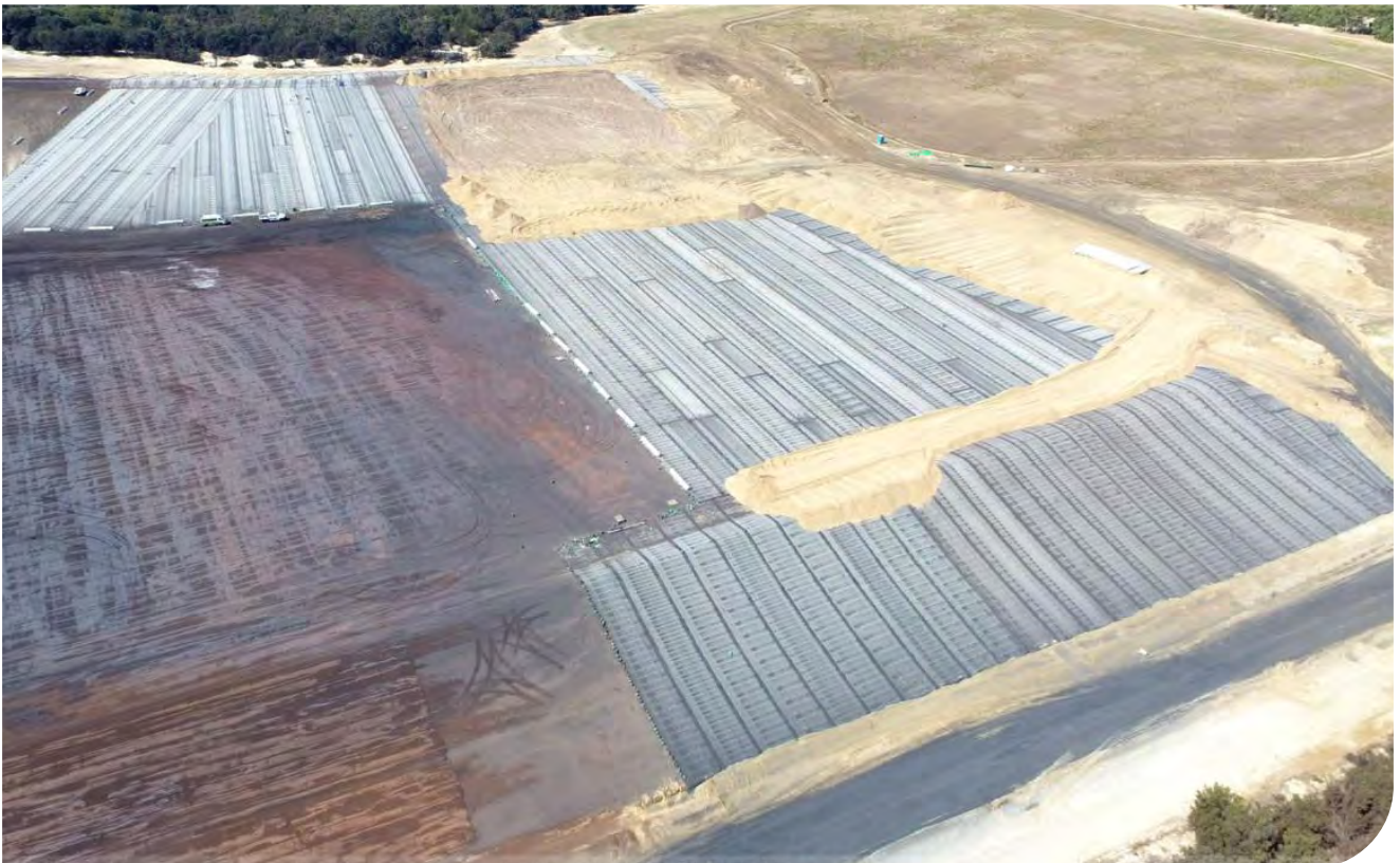
▲ Soil cover layer being applied on a mineral sands waste cap
