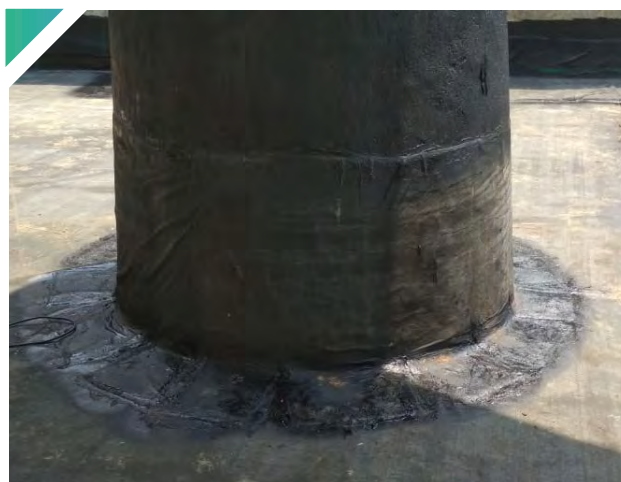
▲ Bonding on concrete footings
