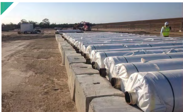
▲ Storage using concrete blocks
