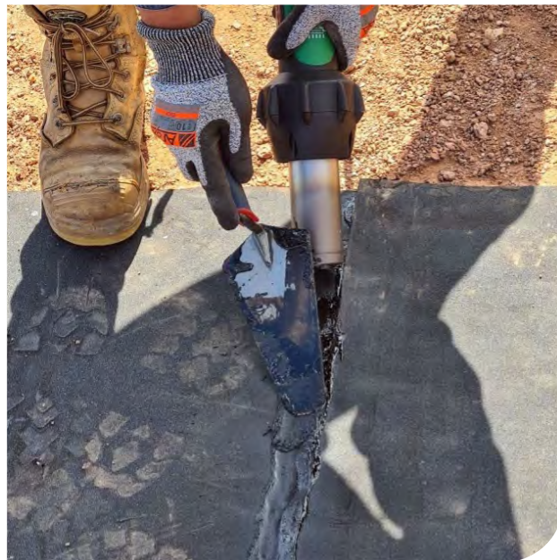
▲ Fillet weld demonstration using the Electron handheld welder and a rounded trowel
