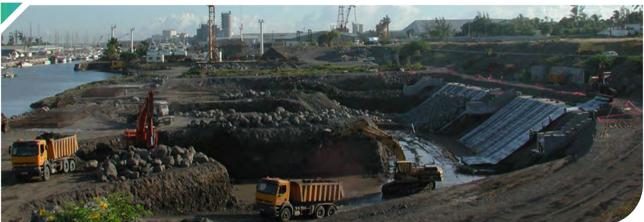
▲ Riprap being installed
