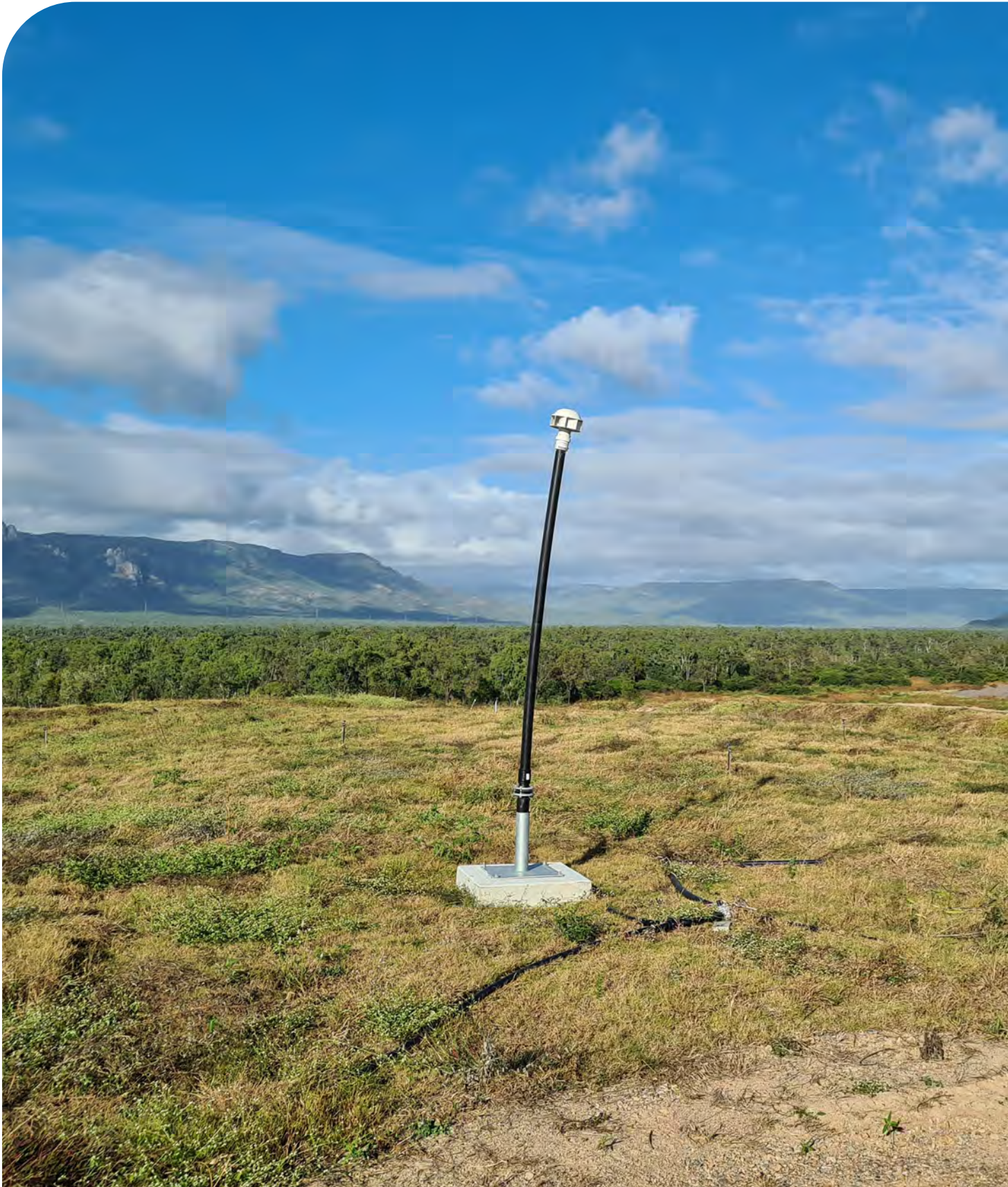
▲ Landfill Cap with gas extraction and soil cover system
