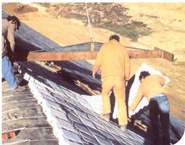
▲ Pre-cast cobblestones, anchored from the crest
