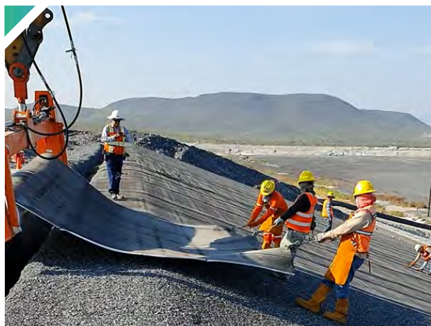
▲ Use of a hydraulic beam on slopes
