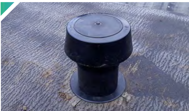
▲ Blowhole installed on Coletanche geomembrane
