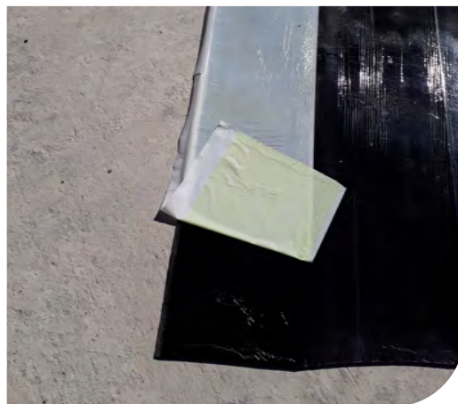
▲ Laying Coletanche overlapping in the flow direction, which required different positions of the PE silicone Film depending on the side of the canal
