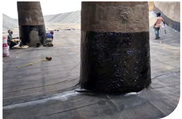
▲ Bonding to pipe and manhole
