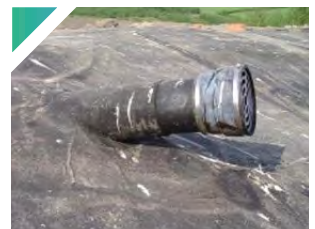
▲ Connection to overhanging pipes
