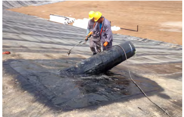
▲ Bonding to pipe and manhole
