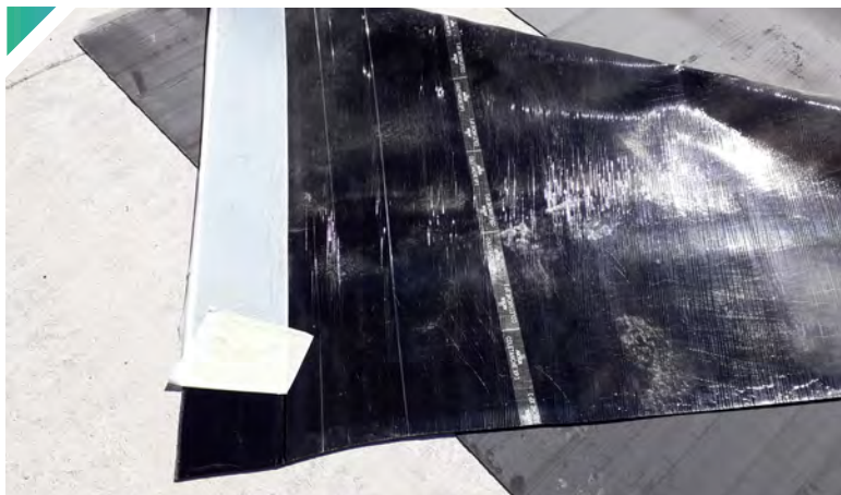
▲ Laying Coletanche overlapping in the flow direction, which required different positions of the PE silicone Film depending on the side of the canal
