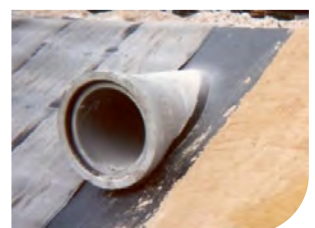
▲ Concrete block and primer coating around a concrete pipe
