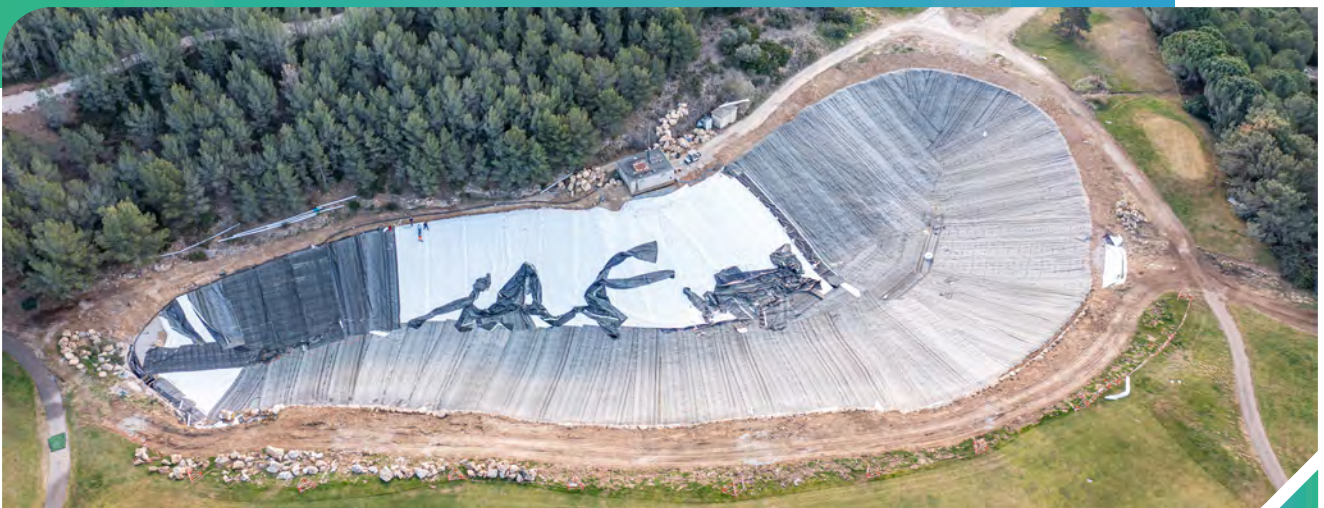
▲ Geomembranes lifted by extreme wind during construction process
