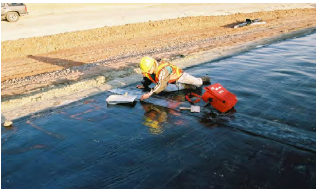
▲ Laying ballast on Coletanche
