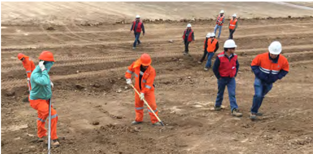
▲ Raking of the subgrade
