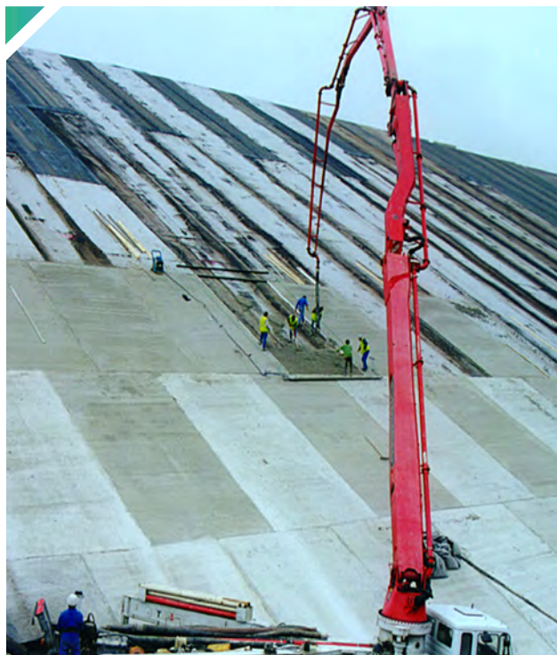
▲ Laying rolled gravel on Coletanche
