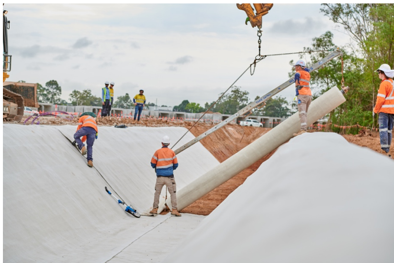
EXCLUSIVE TILTEX B ANTI CRACKING GCCM 80MPa Compressive Strength 16.1MPa* Flexural Strength Up to 5m Wide Rolls
